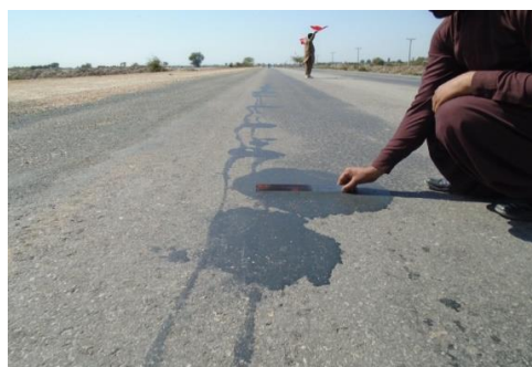
Figure 6. Data recorded on condition survey data Sheet. Photo shows light bleeding
