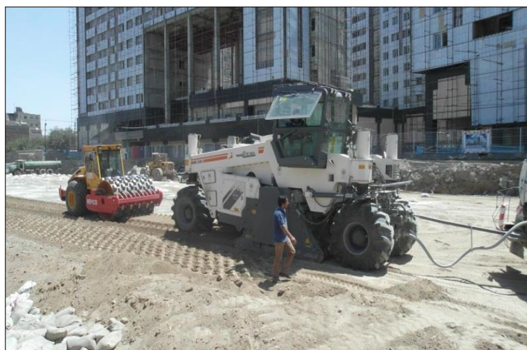
Figure 14. Compaction with sheepfoot roller
