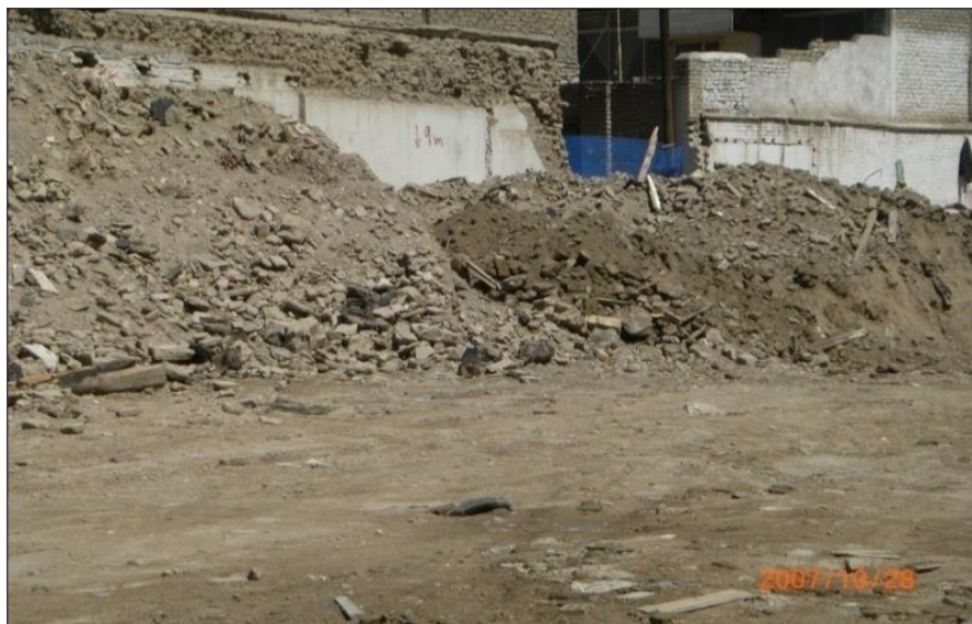
Figure 2. A view of the demolished buildings materials
