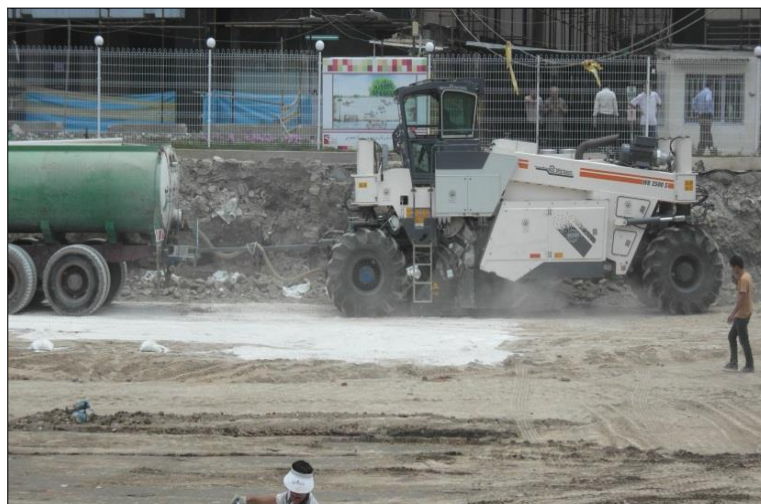
Figure 13. Cement distribution and stabilization with WR4500 equipment
