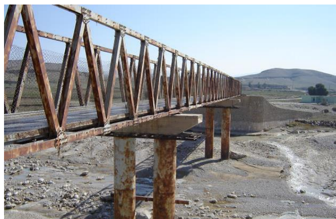
Figure 7. Zulfaqar Bridge on A'la River in the study area
