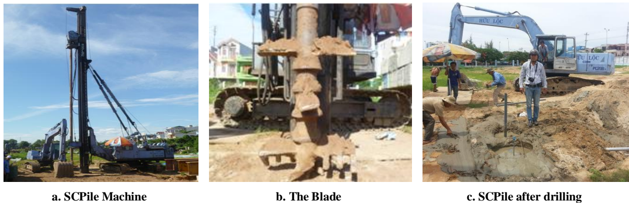
Figure 7. SCpile construction process at si-tu
