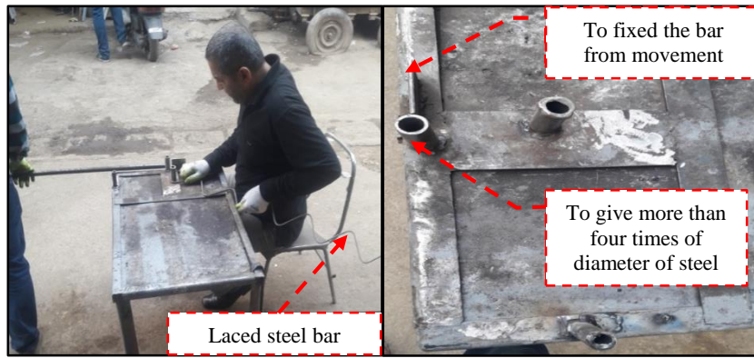
Figure 2. Photograph of Lacing Bars Fabrication
