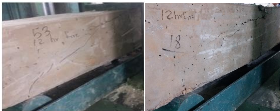
Figure 8. Crack pattern in RC beams
