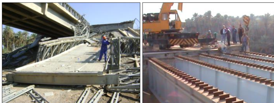
Figure 13. AI SABIYA Bridge
