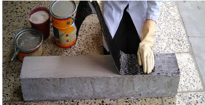
Figure 3. Strengthening beam with carbon fibers
