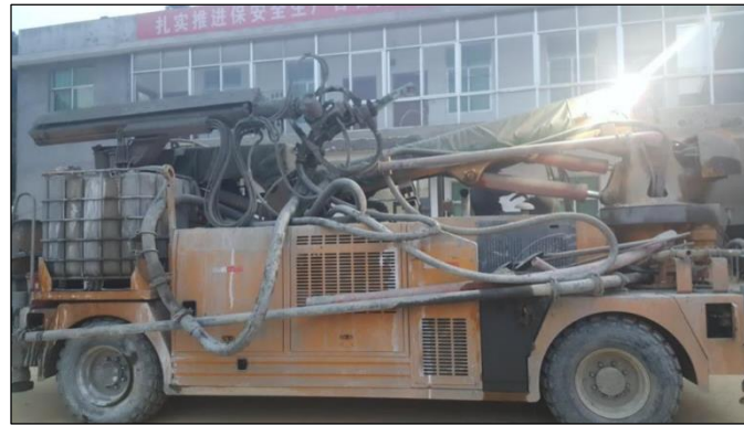
Figure 12. Testing shotcrete vehicle
