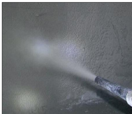
Figure 8. Typical shotcrete spray
