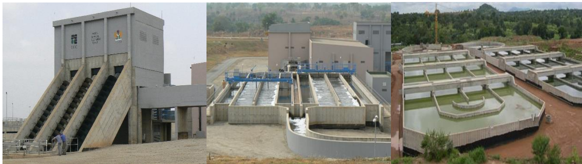
Fig -1: Wupa Wastewater Treatment Plant
