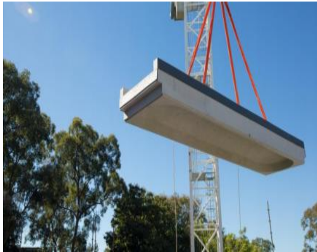
Fig - 15: Meter “geopolymer beam with vaulted soffit being craned into position” [43].
