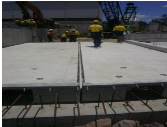
Fig - 14: Installation of prefabricated bridge at Murarrie concrete batching industry [43].
