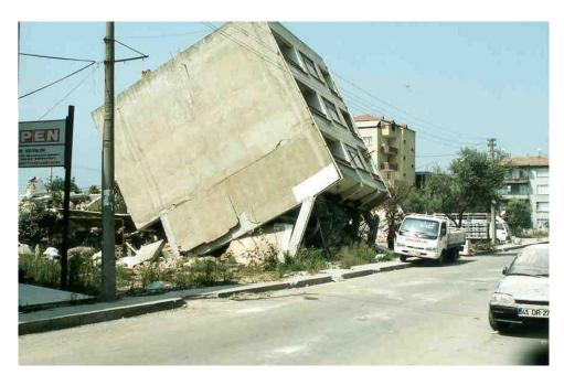
Figure 2. Failure in the form of soft storey mechanism (Kocaeli, 17 August 1999 Marmara earthquake)
