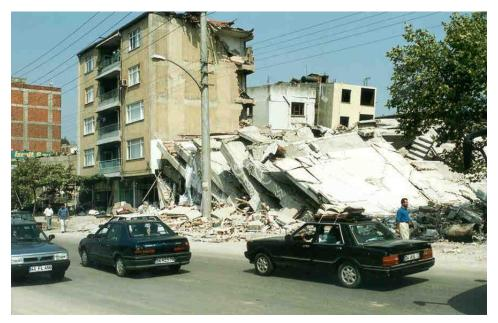
Figure 1. Failure due to lack of lateral stiffness (Derince, 17 August 1999 Marmara earthquake)
