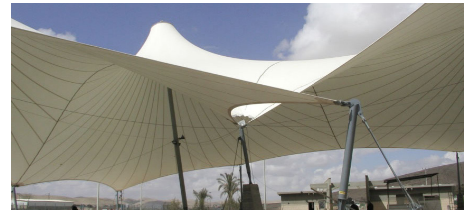
Fig. 21. Tensile structure applied with PTFE
