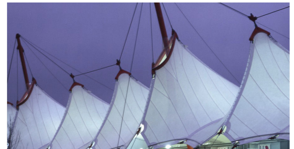
Fig. 22. Tensile structure applied with PVC polyester
