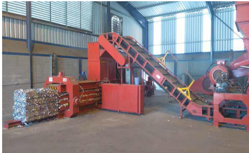
Figure 4.9 Refuse-derived fuel plant at Interwaste recycling hub
