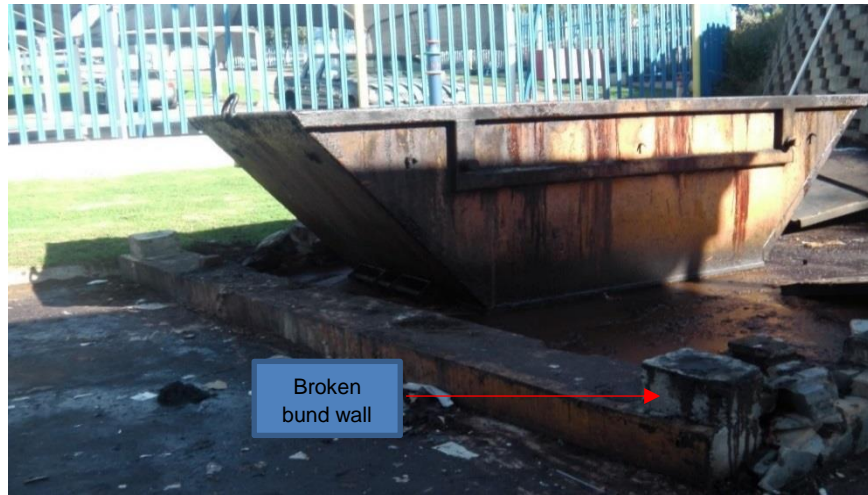
Figure 4.14 Fat skip bund area
