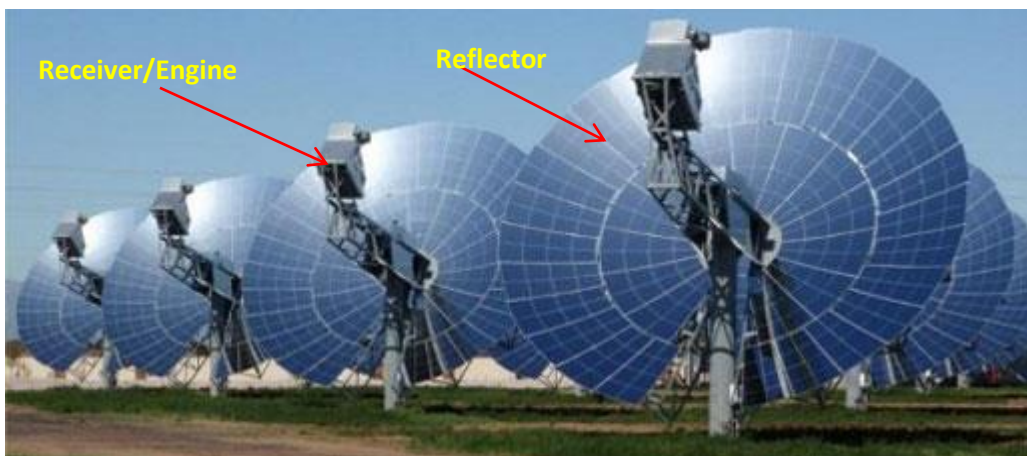
Figure 1.4: Schematic of solar dish system [1.20]
