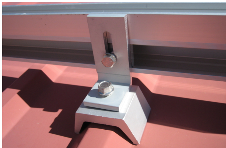
Figure 6: Example of mounting system on sinusoidal, corrugated and trapezoidal metal roofs (Pickerel 2018)
