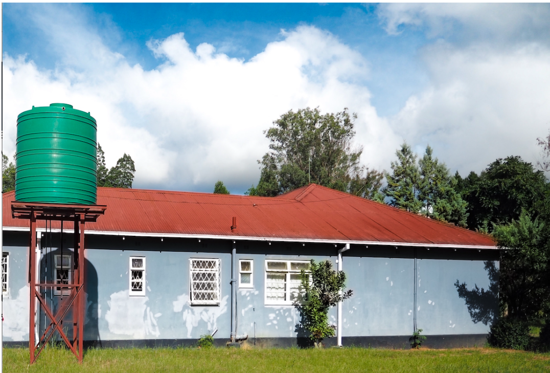
Figure 5: Maternity ward seen from the east
