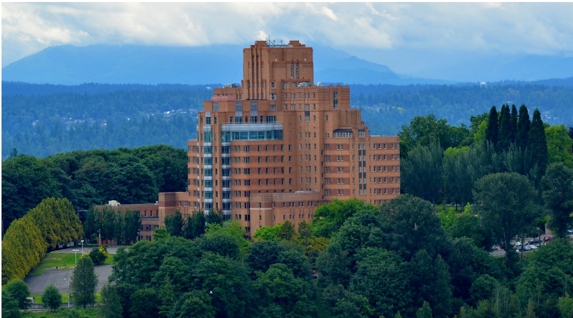
Figure 2.4 Seattle's Pacific Medical Center on Beacon Hill
