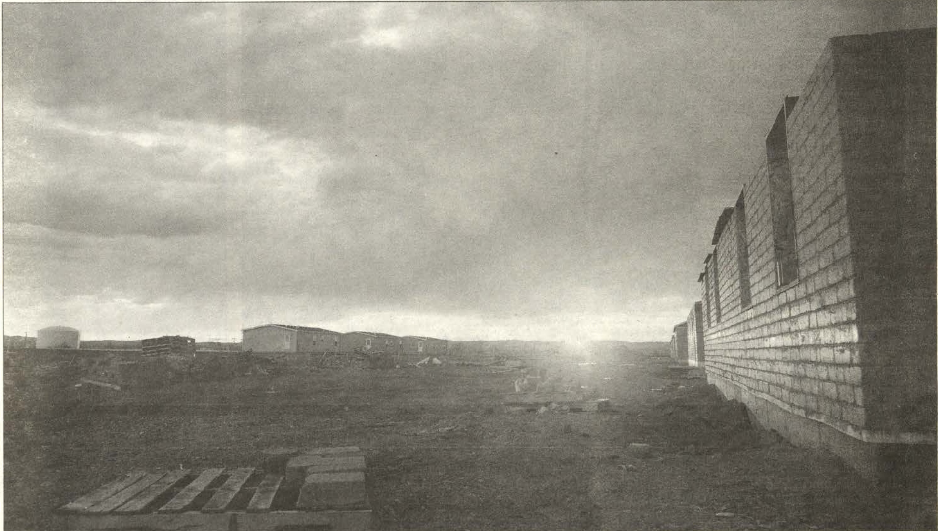
The sun rises over the unfinished Good Earth Lodges in Crow Agency. The project on the Crow reservation was started in 2010 in conjunction with the University of Colorado-Boulder. The team developed large bricks made from materials found on the Crow reservation to build the houses.
