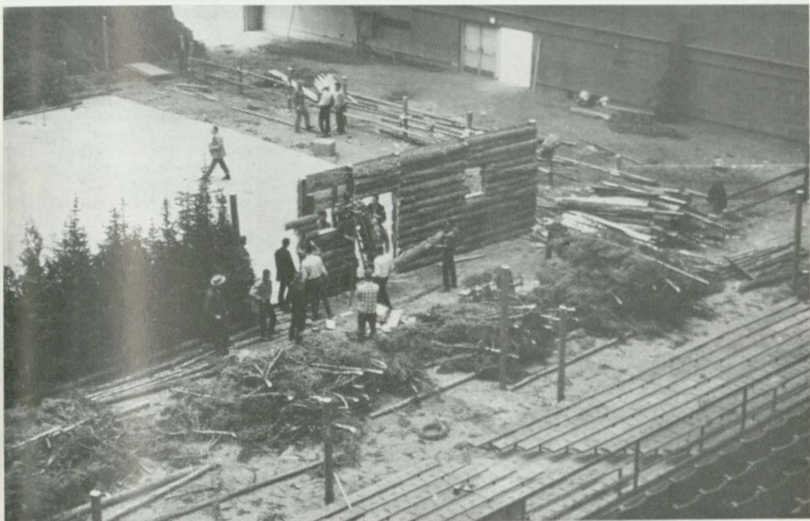
The chow hall begins to take shape in the Field House.
