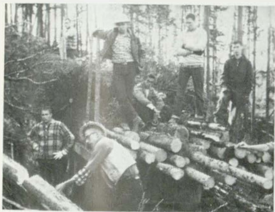
Clearing the road.
