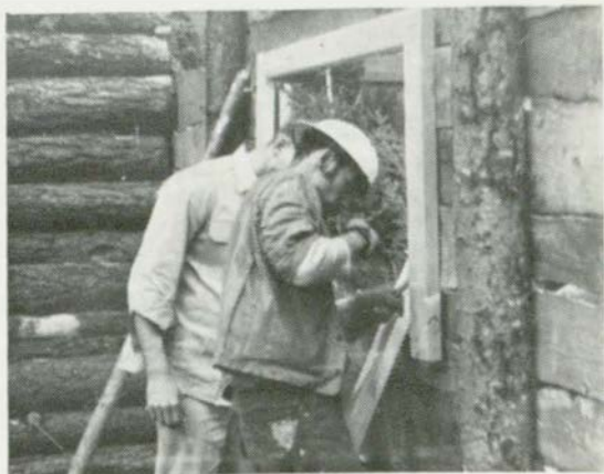
Remick puts the finishing touch on a window.
