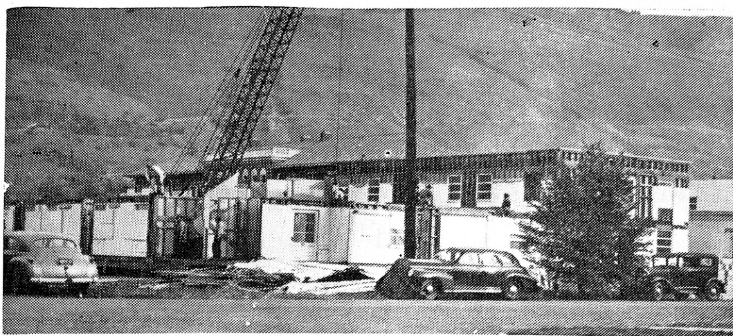
Jumbo hall emerges from prefabricated jigsaw puzzle.
