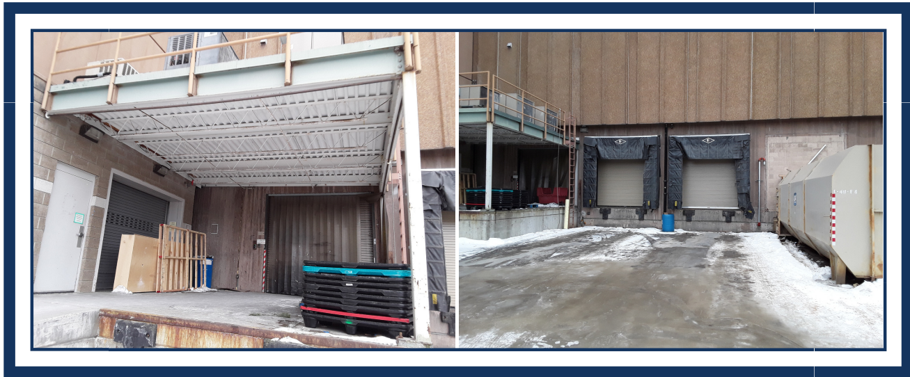
Figure 10. Loading dock roof and doors
