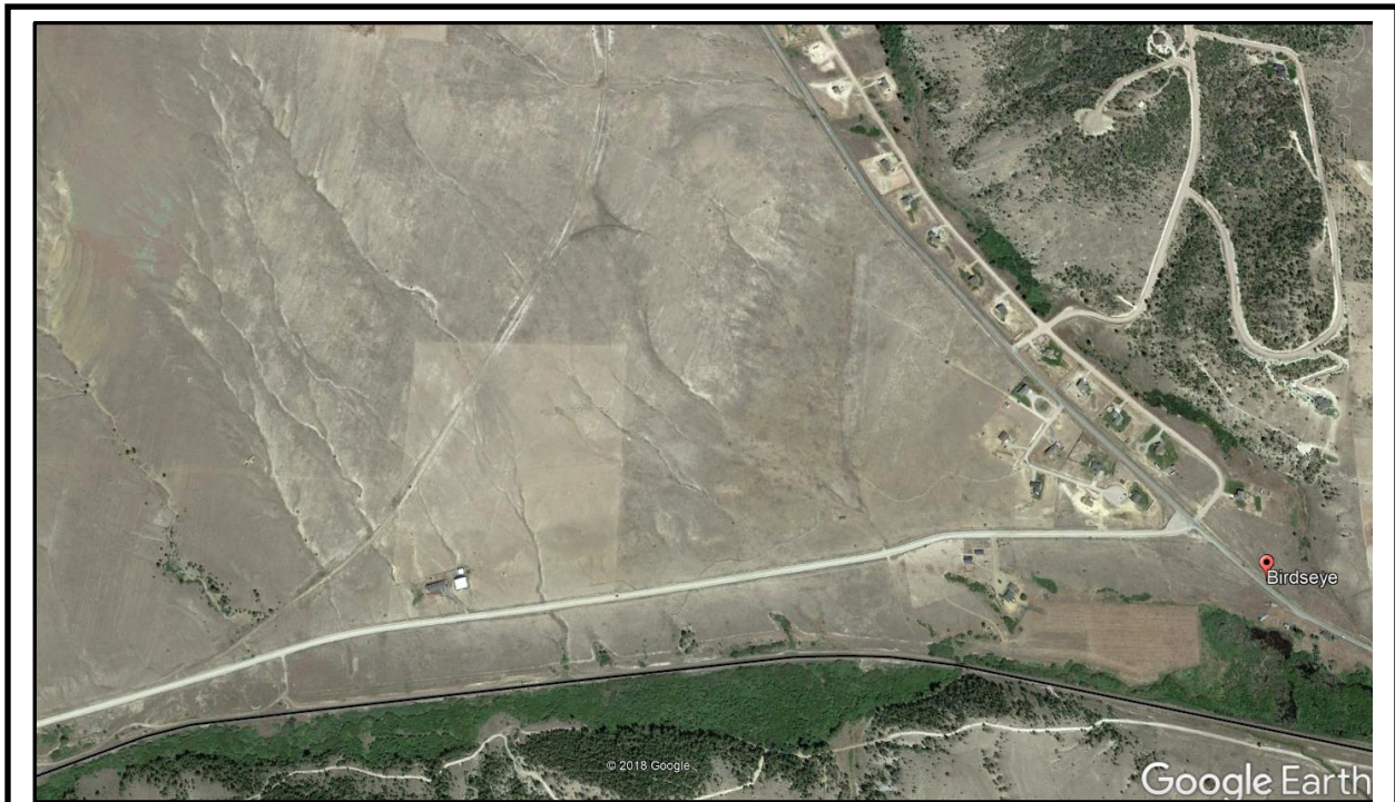
Figure 3. Google Earth View of Birdseye and Clough Junction Area. The 1890's Birdseye settlement was near the red marker labeled Birdseye near the right edge of this view. The abandoned H & N railroad grade is the arcuate feature that trends from the southwest corner of the view (lower left) to the top of the view near the center of the frame. The turning wye with stub siding is visible on the east (right) side of the grade somewhat above the center of the frame. The Birdseye station referenced in the Helena History (2018) website is out of the frame, southeast of the Birdseye marker approximately one third of a mile. Image © 2018 Google.
