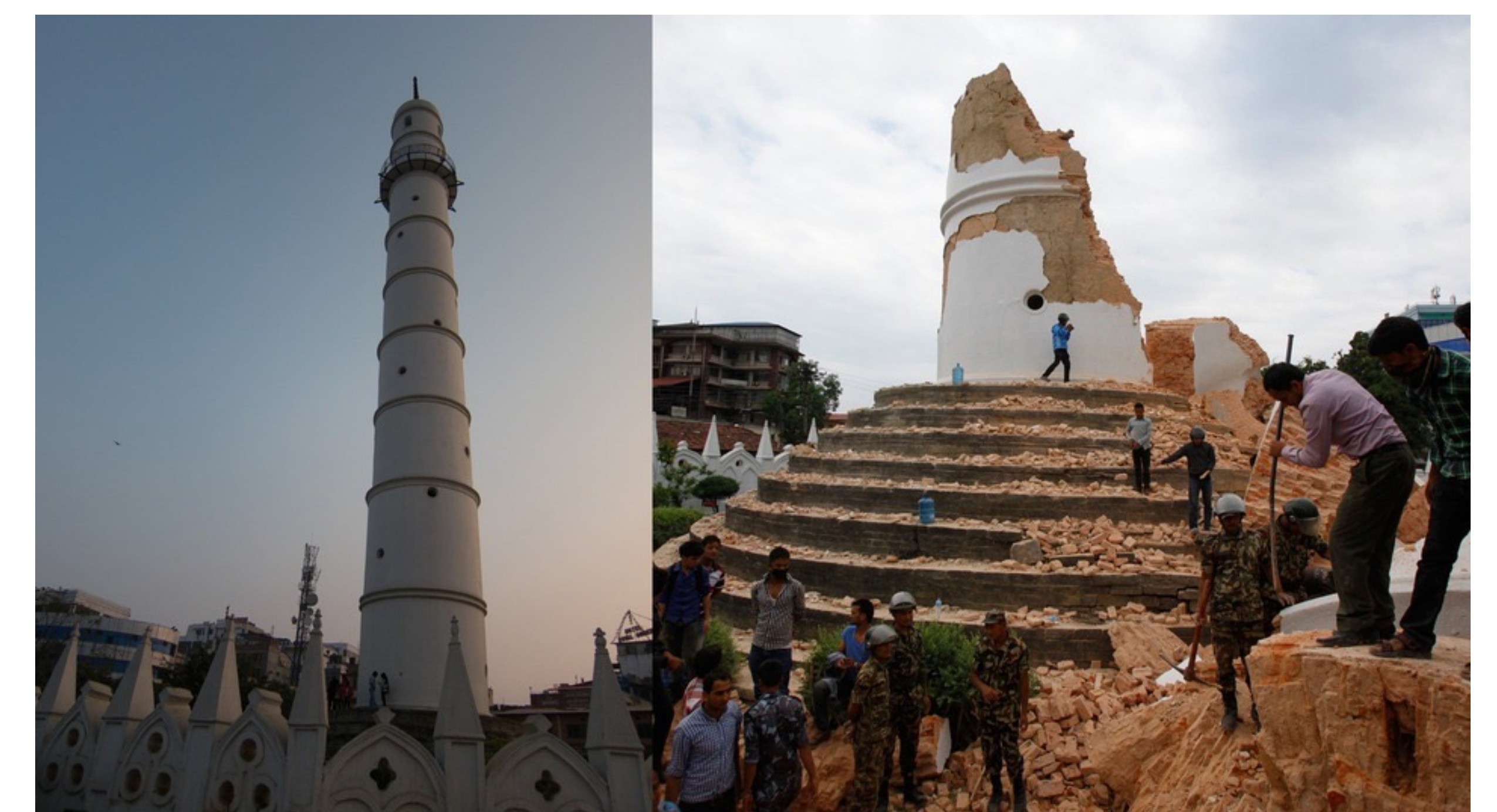
Figure 6: Bhimsen Tower, Kathmandu, before and after the earthquake. Side-by-side courtesy of Mashable; Image: FLICKR, Geoff Stearns; AP, Niranjana Shrestha.
