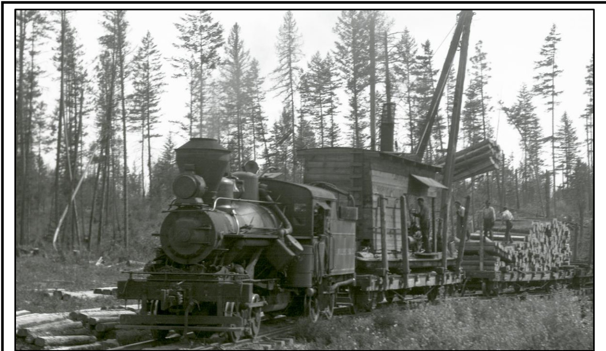
Figure 3. Polleys Lumber Company Locomotive #2 Loading Railroad Ties onto a Flatcar. Ties to be loaded can be seen in the lower left foreground. The “2” is barely visible on the smokebox door even in the original photo. This is MMP photo umt010969 .
