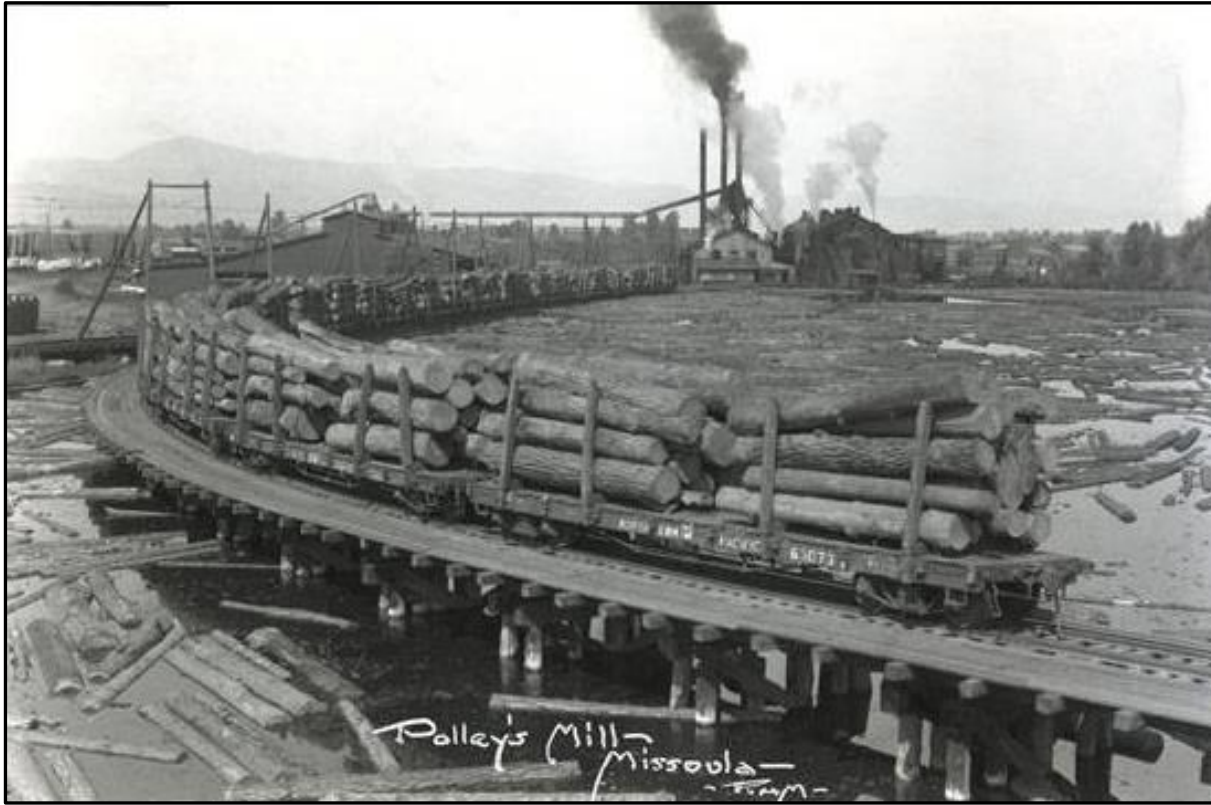
Figure 1. Northern Pacific Rail Cars Loaded with Logs on the Northern Pacific Spur at the Polleys Lumber Company Mill Log Pond. The Northern Pacific spur actually was on a trestle bridge in order to cross the southeast corner of the log pond. The Milwaukee Road spur joins the Northern Pacific spur in the left center of the photo near the trolley wire support with the sloping back brace pole. Other trolley wire supports have similar back bracing. The back bracing can be seen more clearly in umt016885 . This is MMP photo umt010978 .
