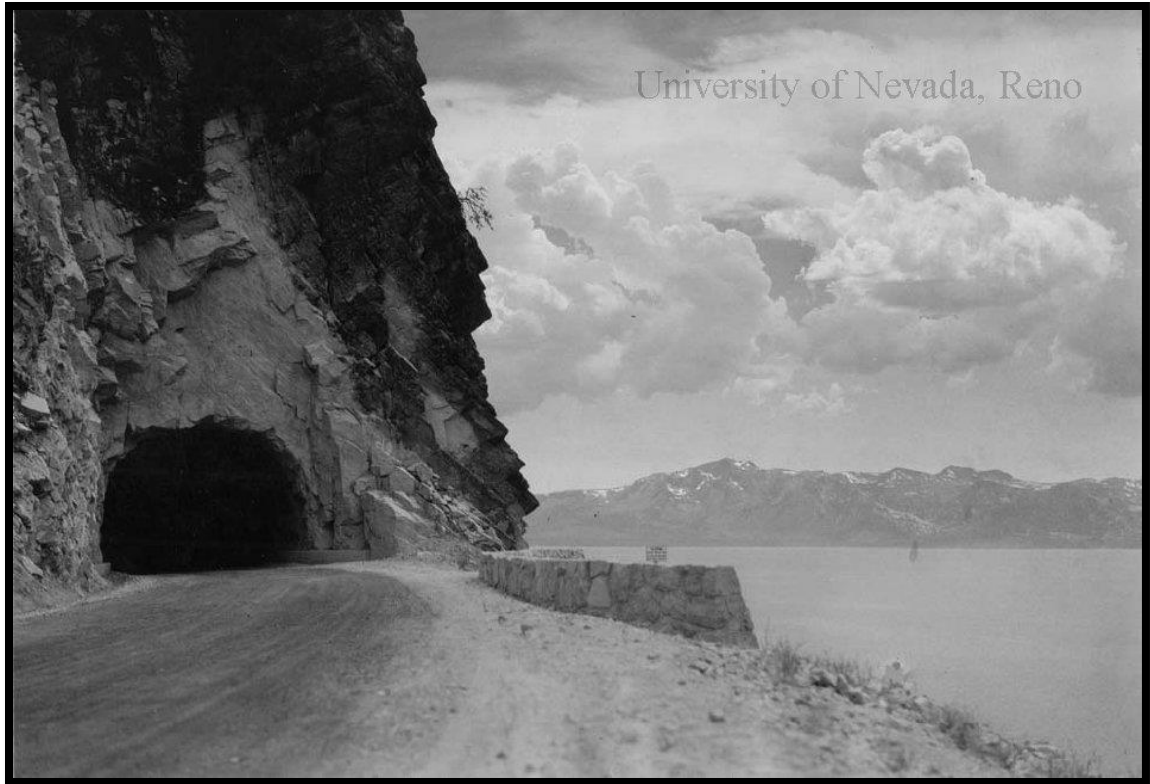
Figure 166. The first tunnel (Herz 1940s).
