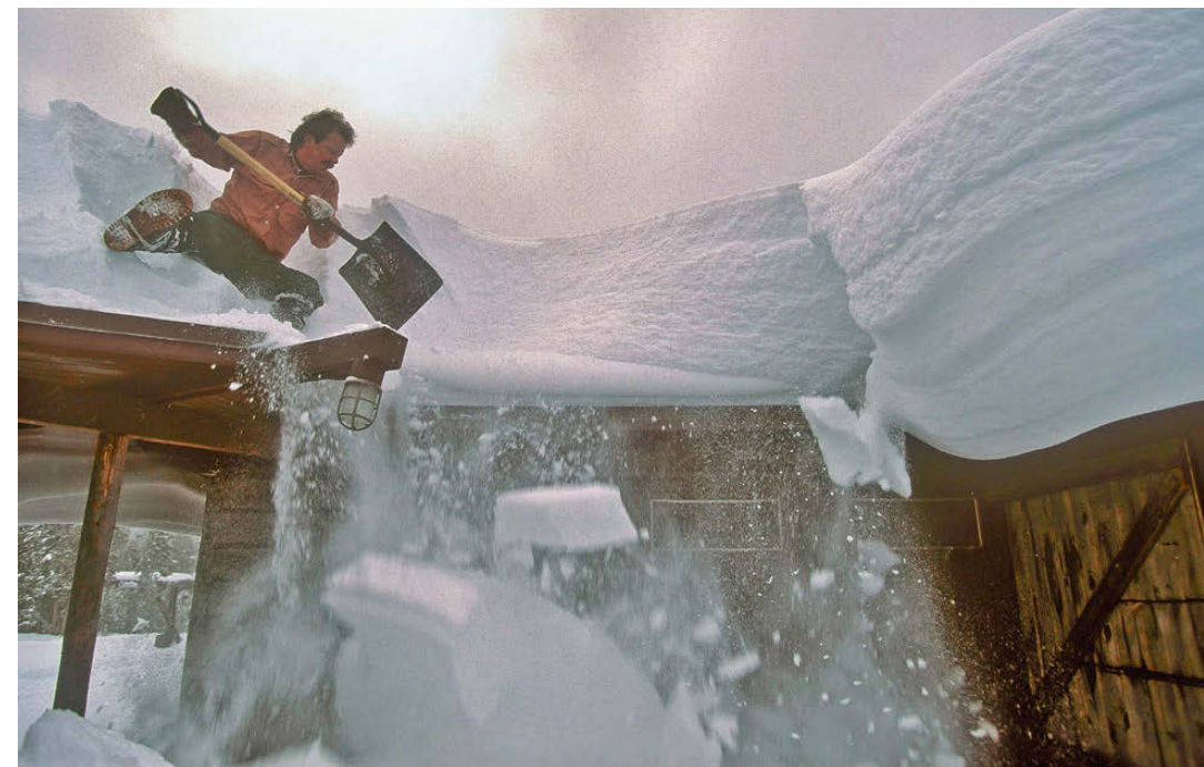
Keeping up with the snow load on the roofs is a never-ending, monumental task. Courtesy of Steve Fuller
