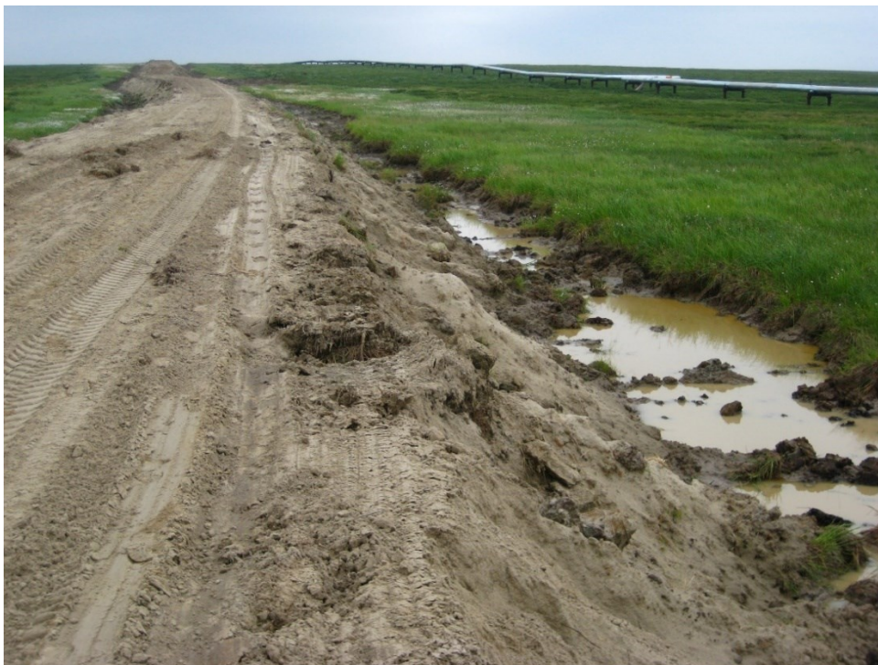
Figure 16. Small, linear features of pooling water adjacent to a road. Pooling is caused by road construction altering the height of the permafrost table and resulting changes in hydrology.
