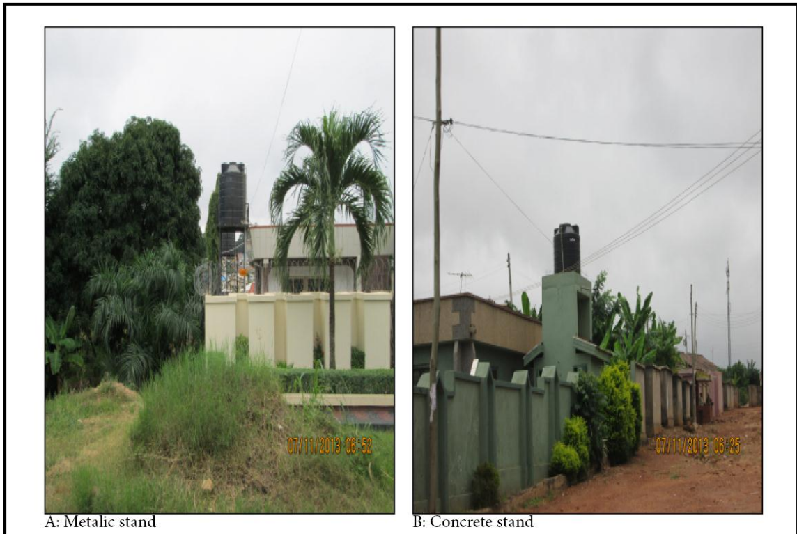
Figure 13: Water storage facility - Overhead tank (Source: Fieldwork, July 2013)
