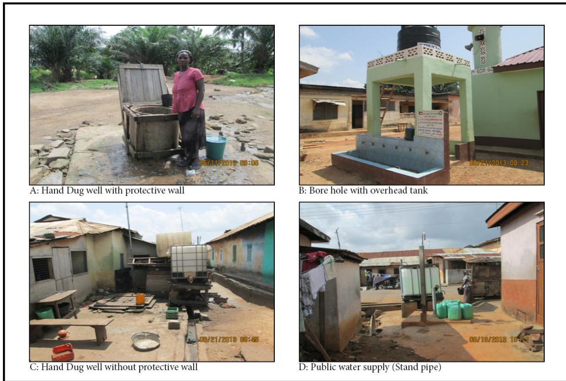
Figure 9: Sources of water supply (Source: Fieldwork, July 2013)
