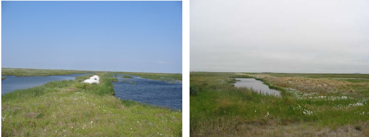
Figure 2. Examples of surface-water ponding adjacent to buried natural gas transportation pipelines.
