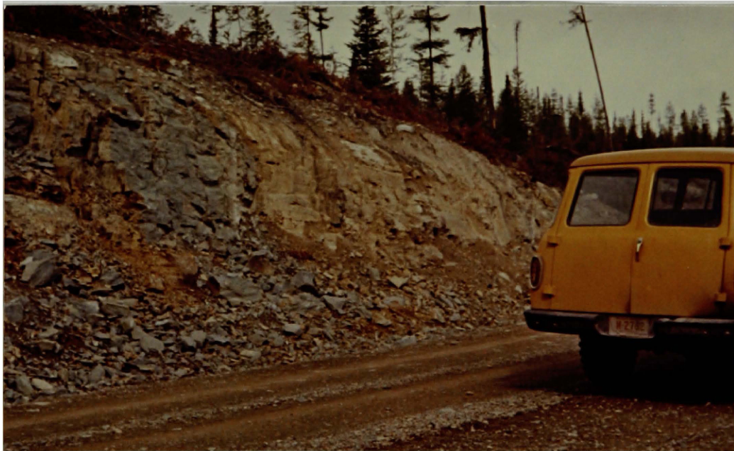
Figure 11. Jointed Siyeh Formation with blocky appearance on Keith Mountain in the eastern part of the area.
