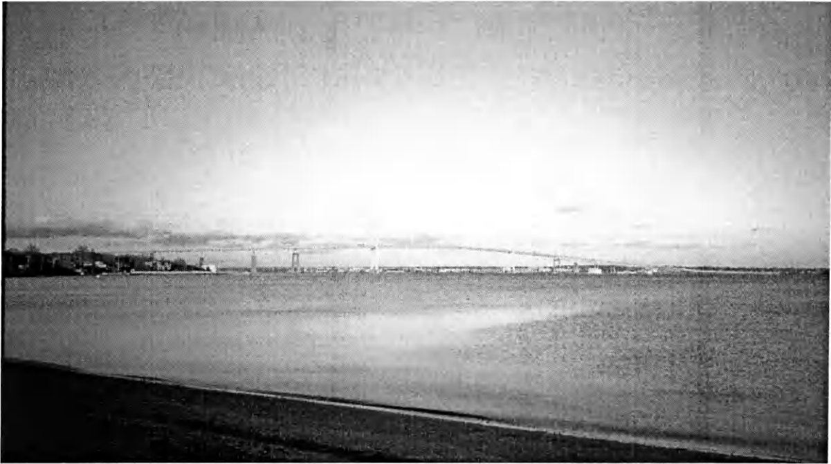
Photo 5: East Passage and The Newport Bridge
