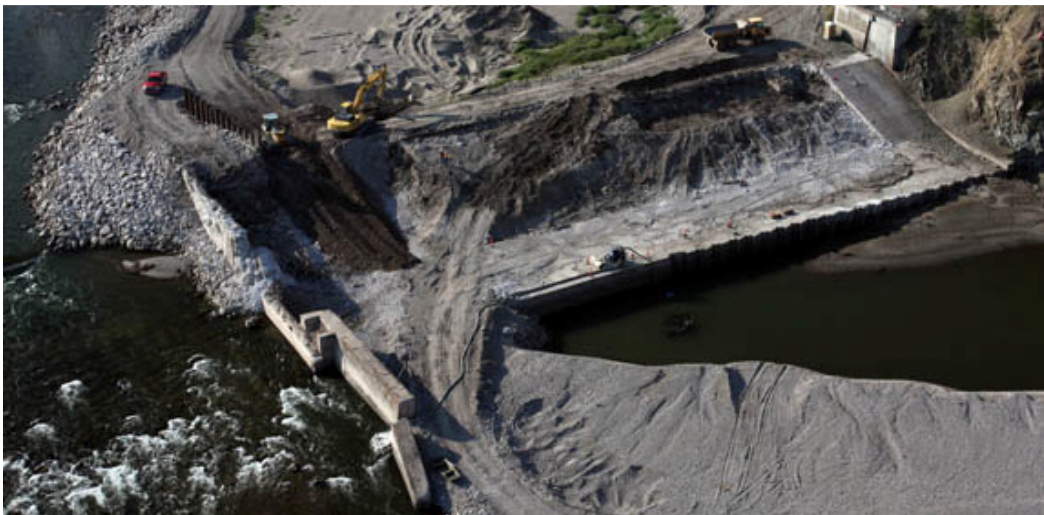
Figure 2.17 Photo taken of the scour hole deposit (bottom left) in the summer of 2008 (looking SSE) (Clark Fork Coalition, 2009).
