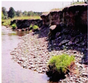
Photo 8: Erosion below Transect 20.
