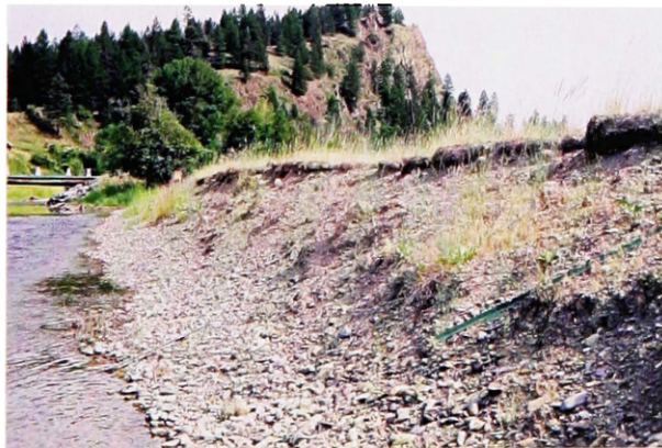
Photo 10: Erosion above Transect 23.
