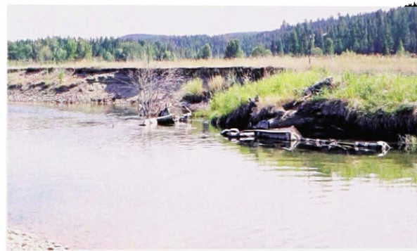
Photo 11: Autobody rip-rap “stabilizing” the streambank below Transect 23.
