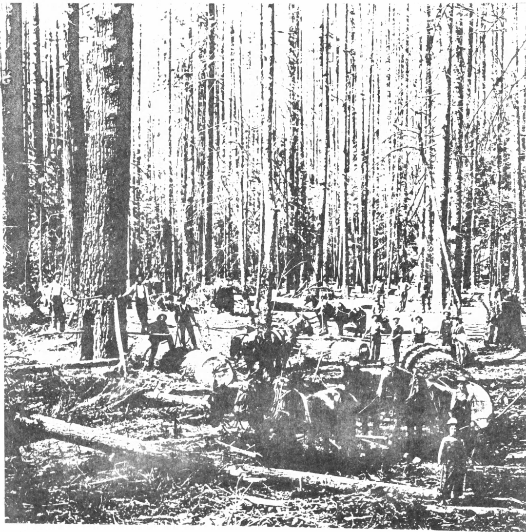
Figure 20. It took a lot of hand labor to change the face of the land, even in smaller timber, but fervent work eventually brought it about. (Meiser Photo)
