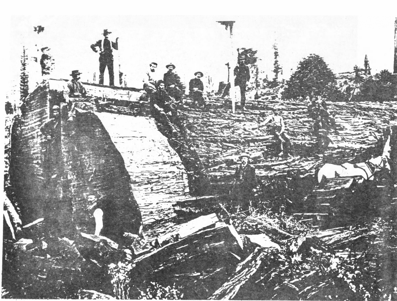
Figure 34. This nineteen foot diameter redwood is being made into railroad ties and shingle bolts. (Meiser Photo, 1905)
