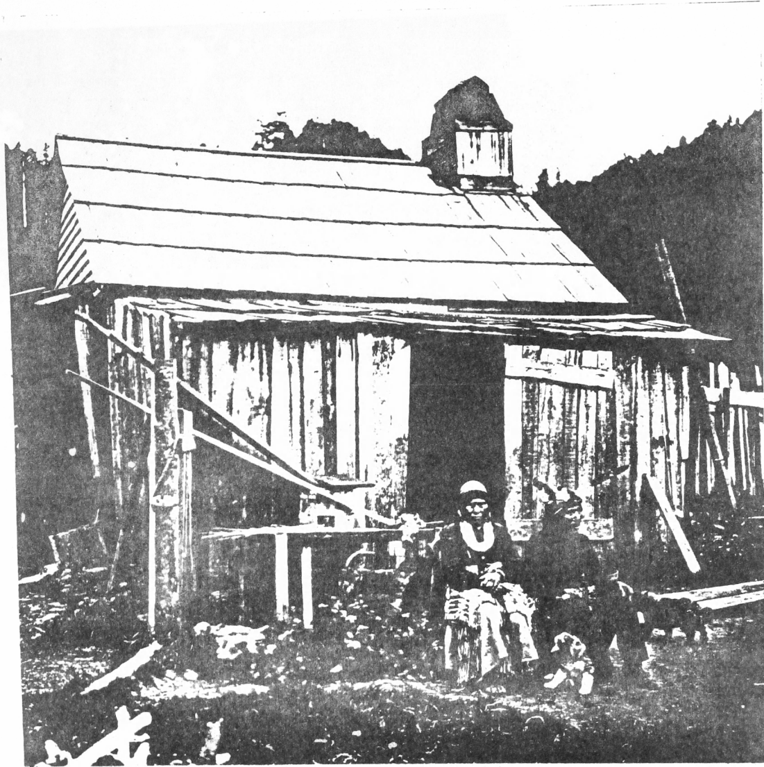
Figure 11. Indian Jim and squaw in front of their house on Cushon Creek. Hupas built houses of split and hewn planks. Farther south, the planks gave way to crudely made bark homes which were hardly more than a conical pile of bark. 8 (Meiser Photo)
