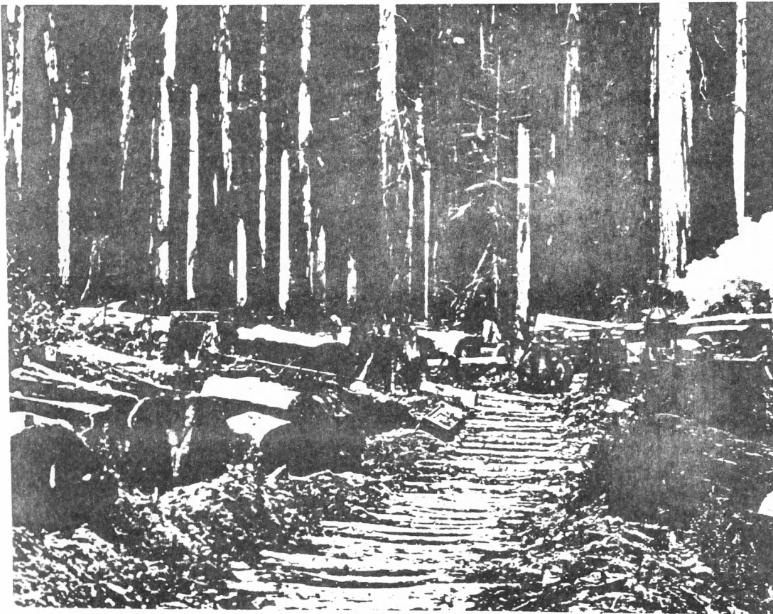
Figure 47. This type corduroy road was common in both oxen and steam donkey operations. Note steam donkey working at the end of this road. (Meiser Photo)
