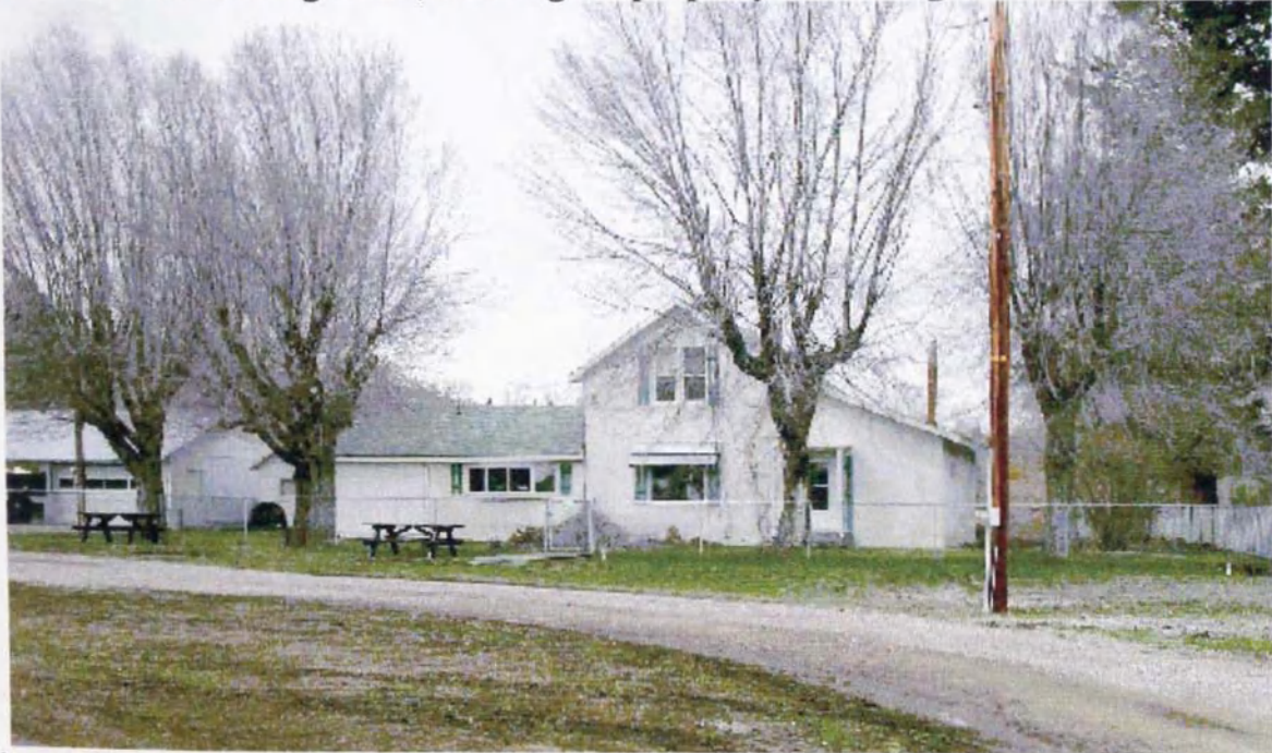
Figure S2 – View of main house (south side) looking north-northwest; garage portion of the garage/storage structure visible on left; ‘L’ turn in main access road in foreground as is area of current parking (lower left).
