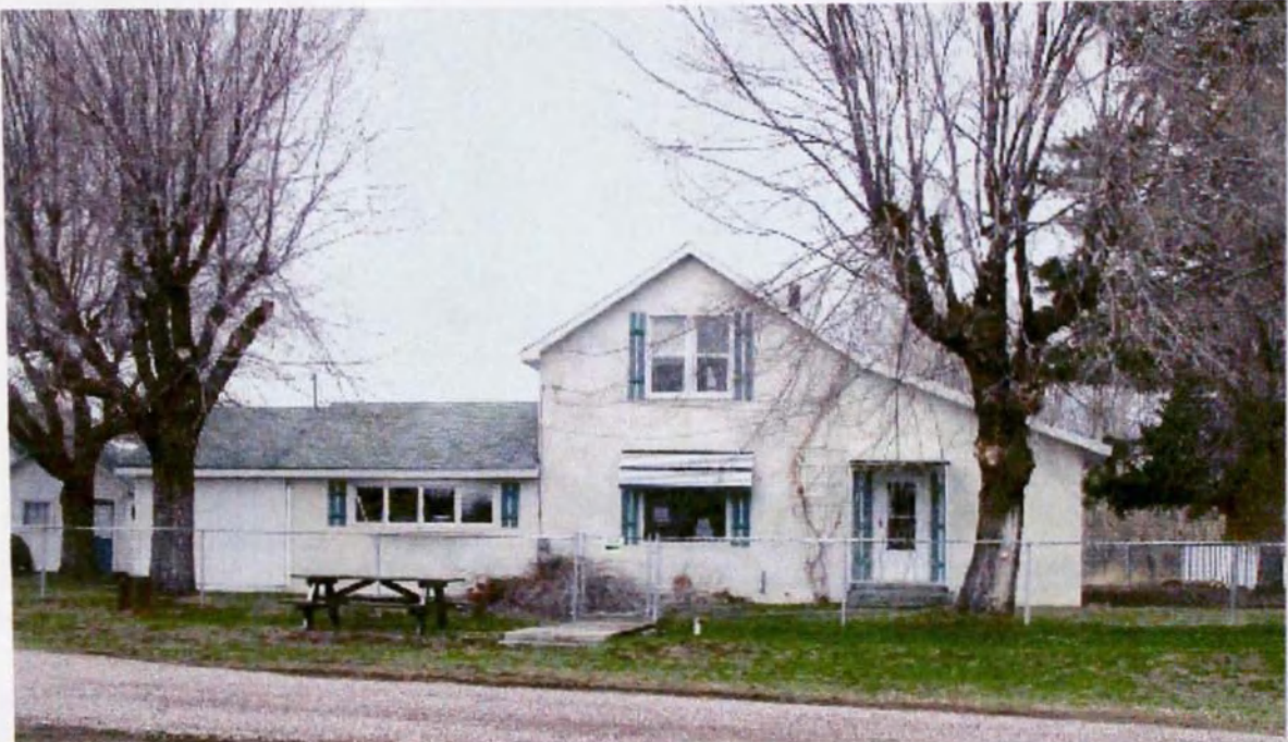
Figure S1 – Front view (south side) of the main house structure, looking north; main entrance drive in foreground; east edge of property line on right-hand side.
