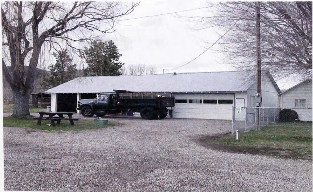
Figure S7 – Front view (south side) of garage/storage shed, looking northwest; garage portion of structure on right with door down; circular driveway evident in foreground; calving shed in background on left.
