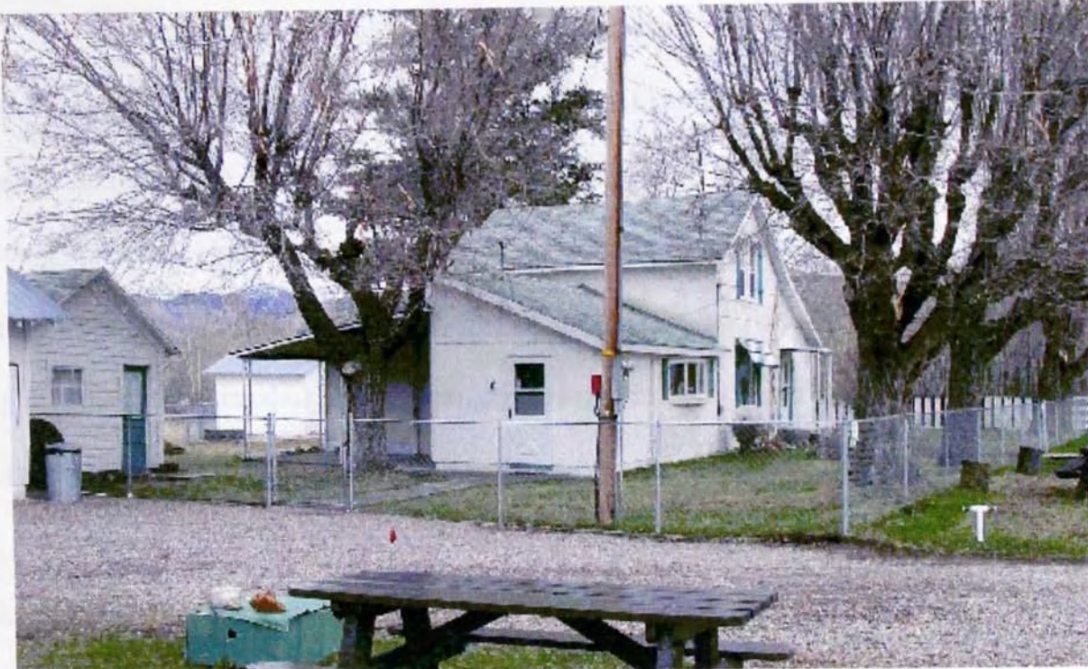
Figure S3 – View of main house (southwest corner) looking northeast; storage structure on left-hand side; garden shed in rear of house.
