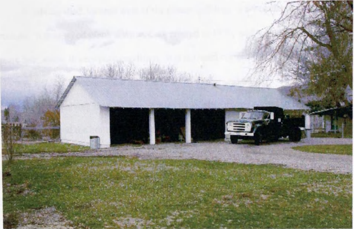
Figure S6 – Front view (south side) of the garage/storage shed, looking north-northeast with the storage portion prominent; truck blocking garage portion; circular driveway section in foreground and right; field access road remnant on left.
