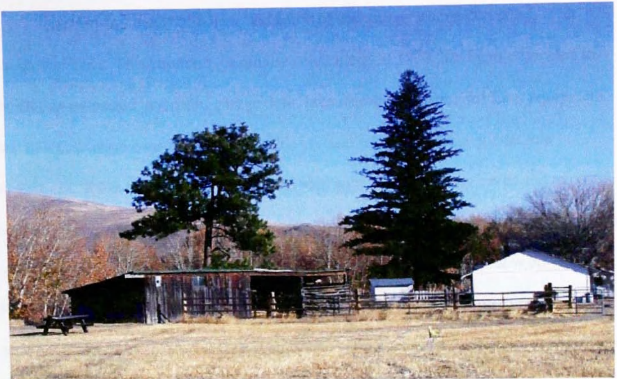
Figure S9 – View of the calving shed and wood corral feature, looking east; garden shed and garage/storage structure in background on right; location of structures follows natural ‘bowl’ shape of slope.
