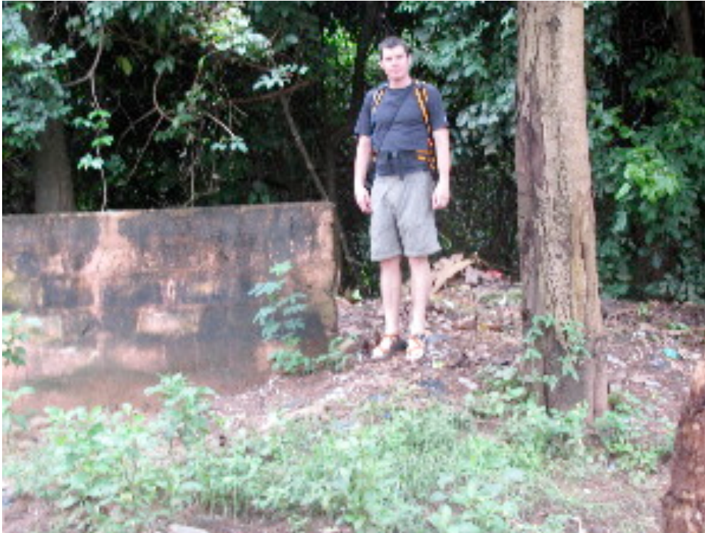
Figure 24. Author adjacent to the lowest existing point of the Forêt Sacrée de Kpassé's protecting wall
