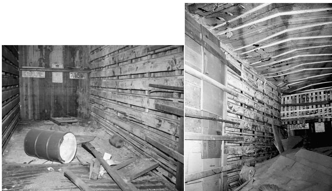
Figure 3.5. Interior shots of both ends of the Area 200 boxcar that derailed in Montana. Note in the right-hand photo evidence of the car being on its side exists in the deformed ceiling supports (from www.hanford.gov ).
