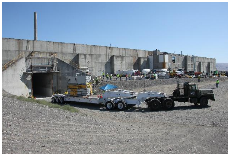
Figure 3.3. Upper Panel: Area 200 West U Canyon Interior view. Lower Panel: Truck removing a waste tank from the exterior of U Canyon. (Retrieved from http://www.hanford.gov/c.cfm/photogallery/imgView.cfm/Recovery/CHPRC-0900540.10%20Attachment%201%20Photo%2013%20U%20Plant%20Canyon%20with%20equipment%20on%20deck.JPG on 4/26/13).
