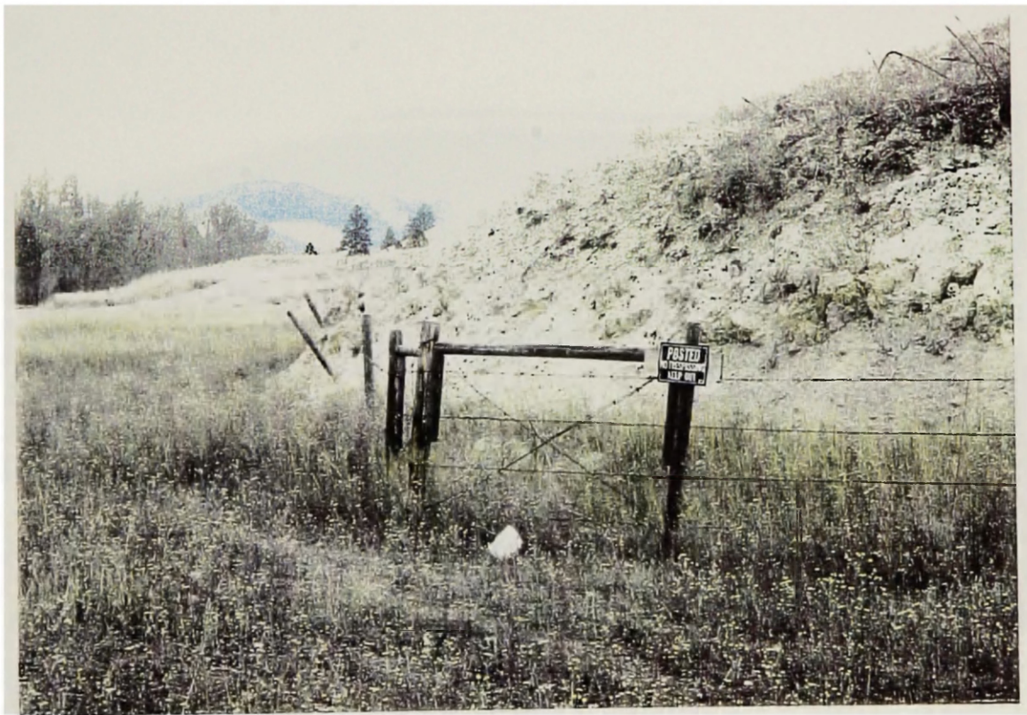
Figure 10: Toe of active landslide
