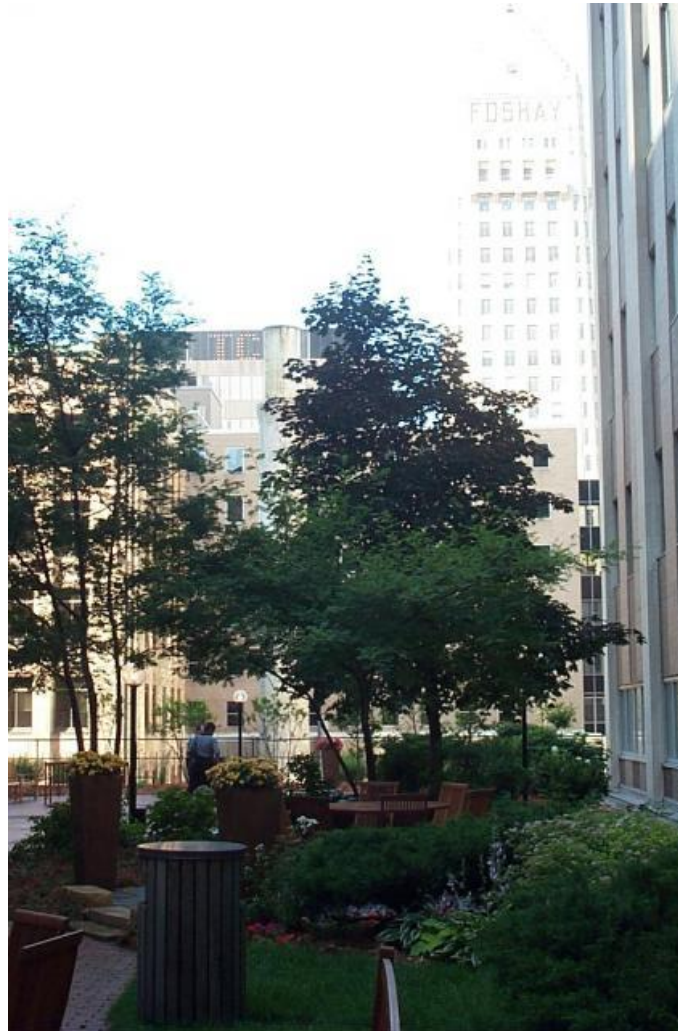
Figure 1: An intensive green roof atop Crowne Plaza Hotel, Minneapolis, MN. Photo via www.mngreenroofs.org .
