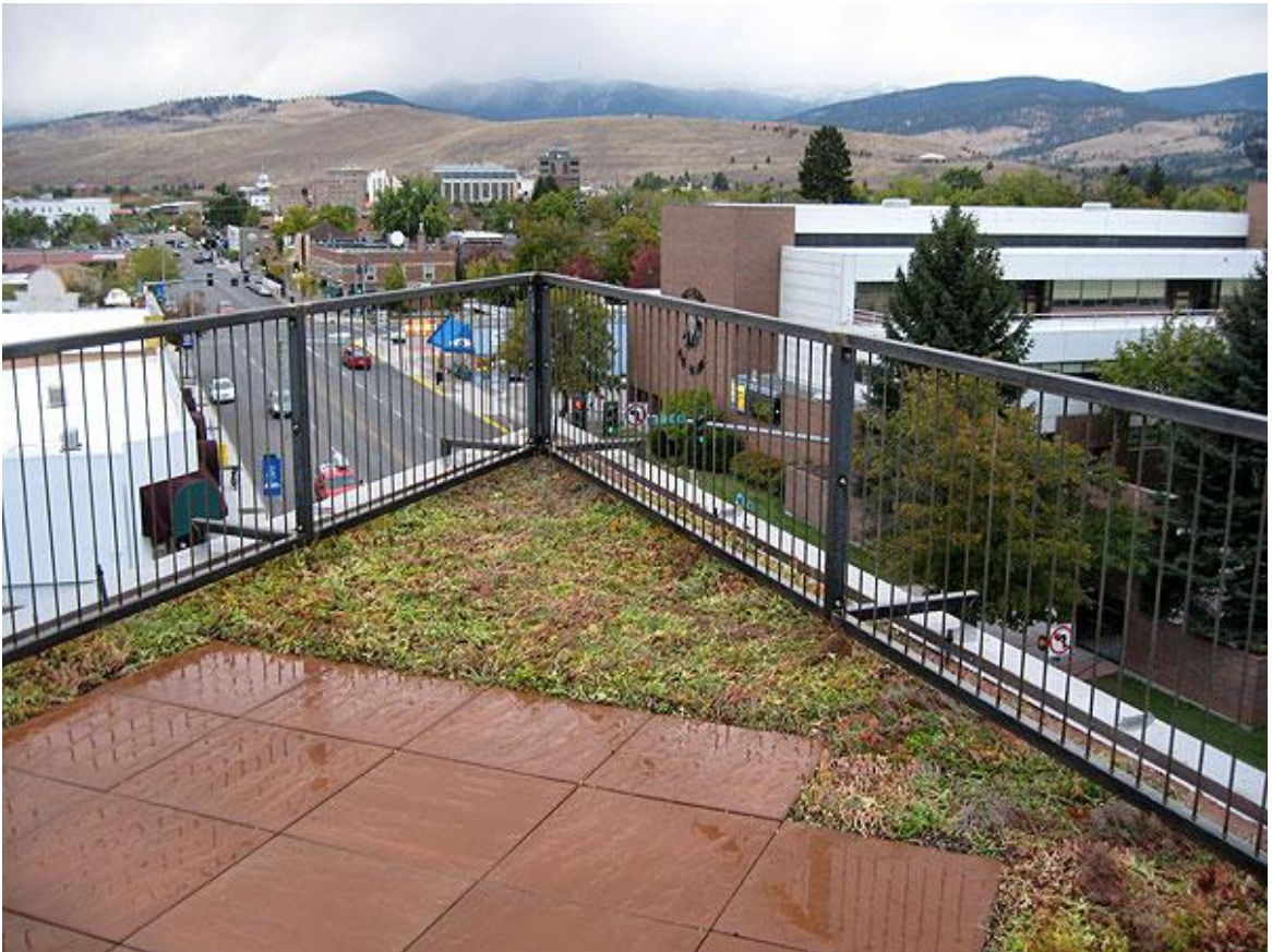
Figure 2: An extensive green roof and hardscape atop the “Corner” 5-story Higgins St. condominium complex. Photo provided courtesy of Eric Hefty, Missoula architect and developer.
