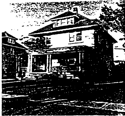
Figure 4. - Company Officers Quarters, Buildings T-28, 29, 31, 32
