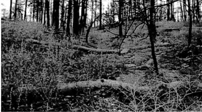
Figure 1: Straw wattles installed on a burned hillslope.
