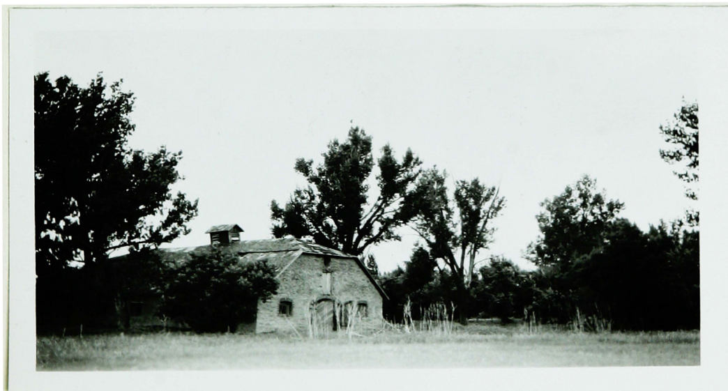
North end of the barn. Built in 1884, this has been called the first stone barn erected in the Northwestern range country.
