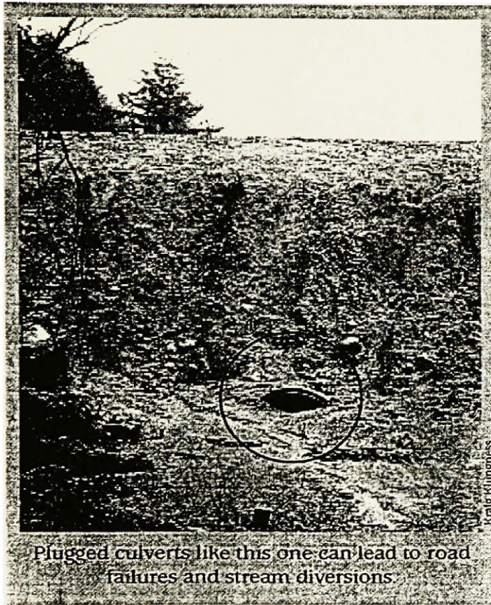
Figure 6. Disfunctional culvert.
