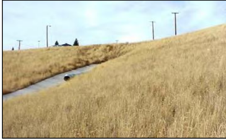
Figure 5-6. West Missoula Gulch after remediation (U.S. EPA 2004)
