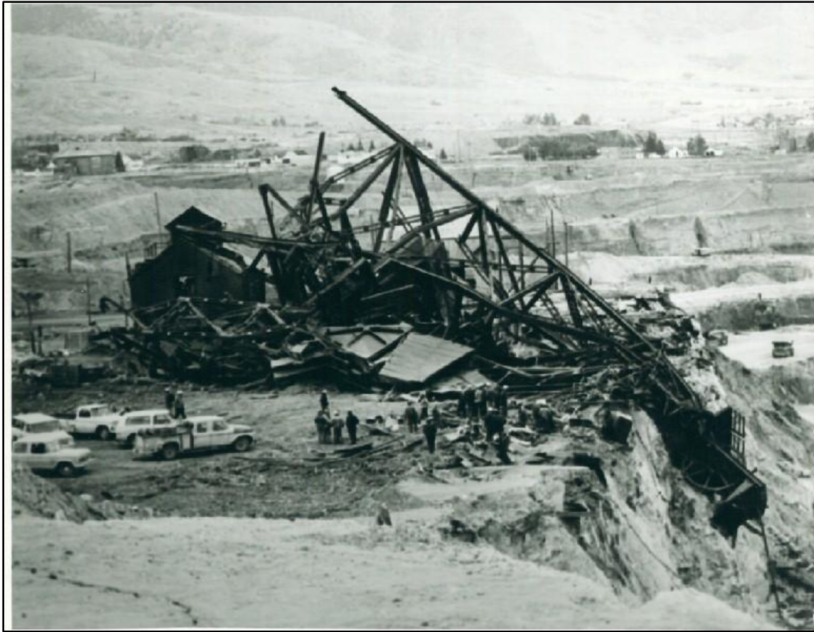
Figure 3-1. Destruction of a Gallows Frame in Butte (Butte-Silver Bow Public Archives Photo Collection 2010)
