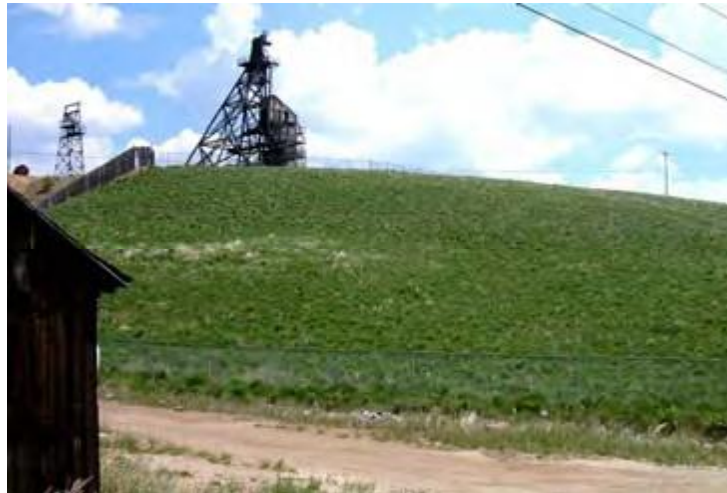
Figure 5-3. Lexington Mine after Remediation (U.S. EPA 2004)
