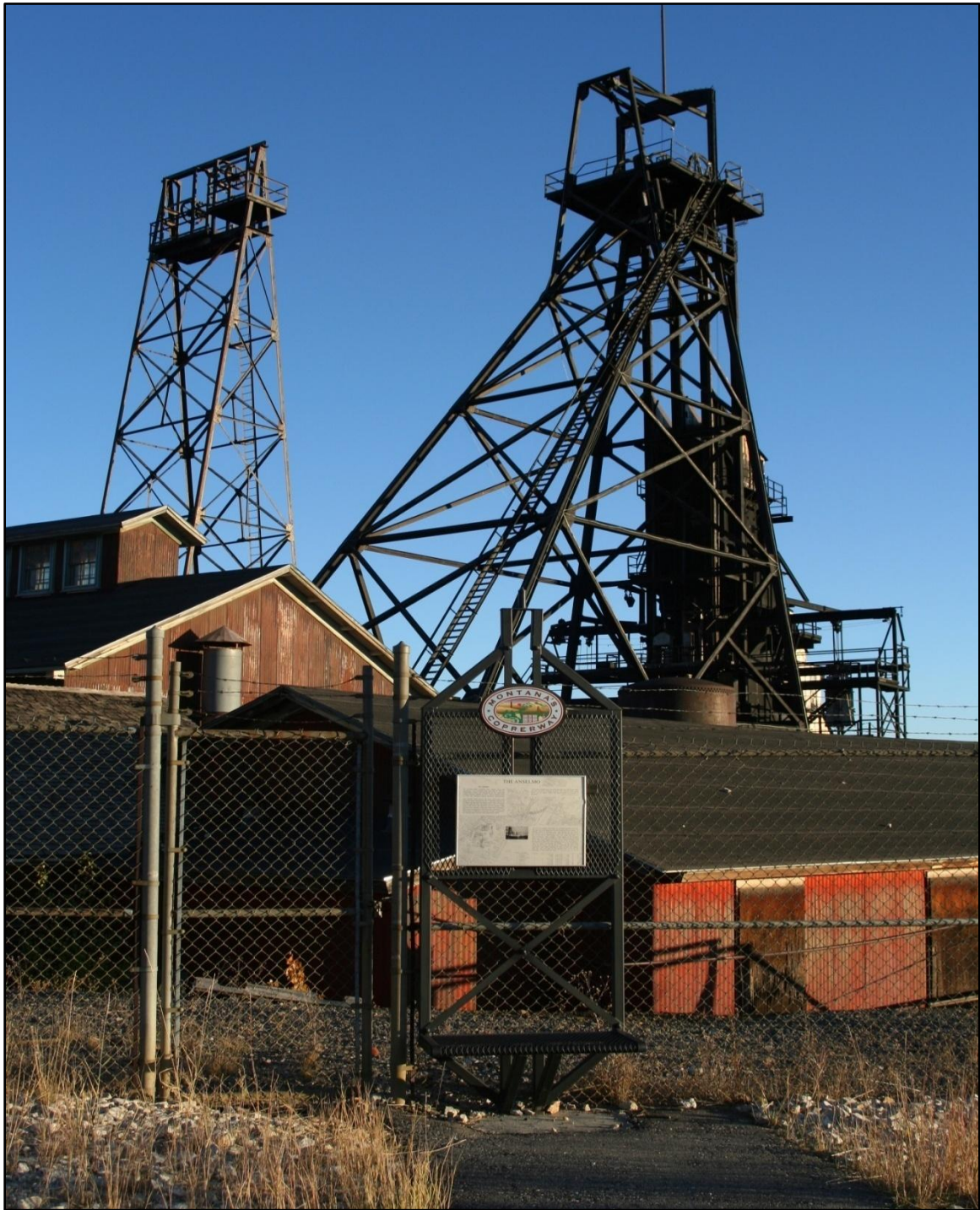
Figure 6-2. Anselmo Mine Yard (Photo by Author)
