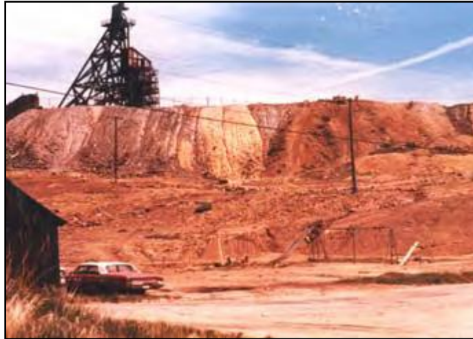
Figure 5-2. Lexington Mine before Remediation (U.S. EPA 2004)
