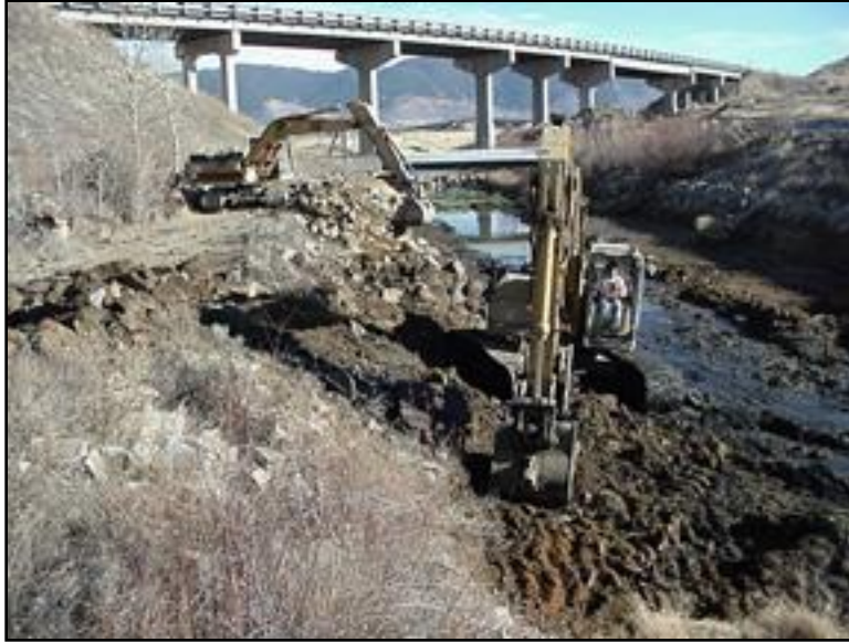
Figure 5-8. Removal of Streamside Tailings (CTEC 2009)
