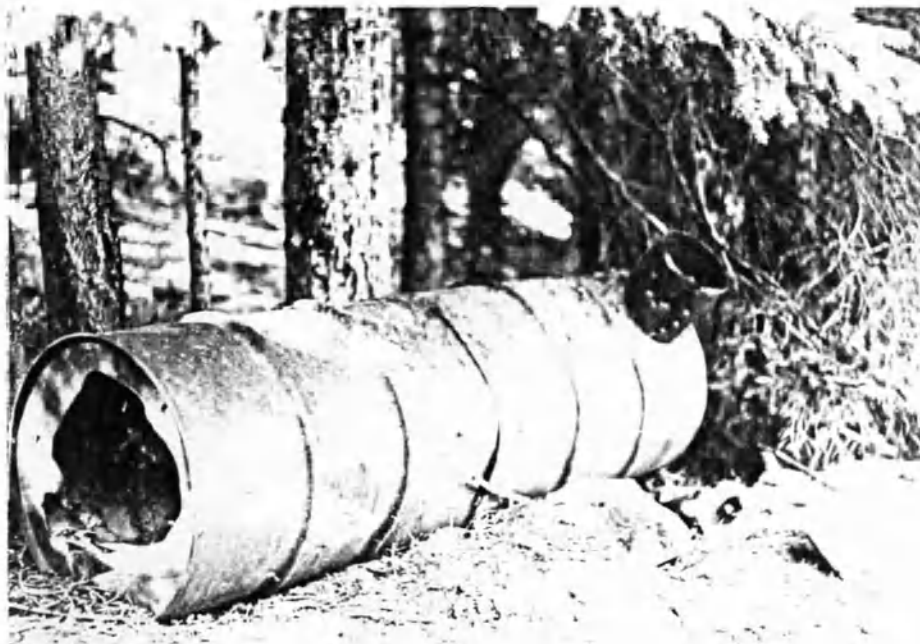
Figure 41: A handmade version of a metal container (Figure 32) used to process ore at the Mountain View mill. It represents low replacement cost.
