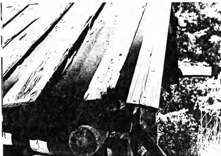
Figure 97: An example of a plank style roof. Notice the tar paper beneath the planks.
