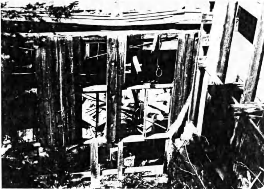
Figure 82: A view into the Mussingbrod mill. The photograph show piles of debris and refuse scattered on the floor
