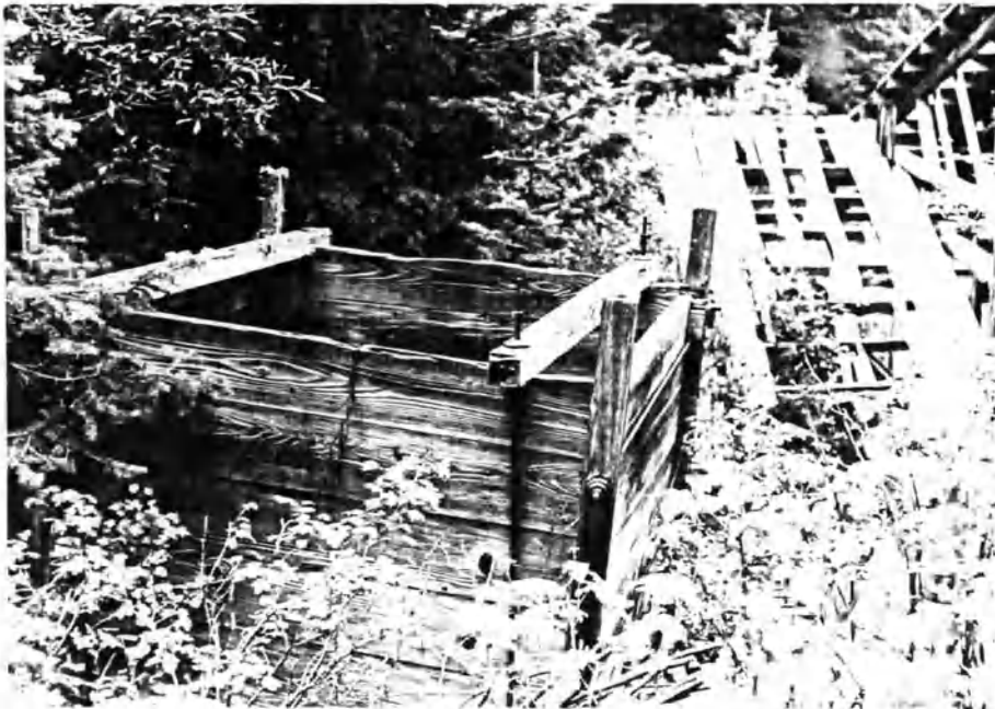
Figure 37: A wooden ore box near the Mountain View mill.
