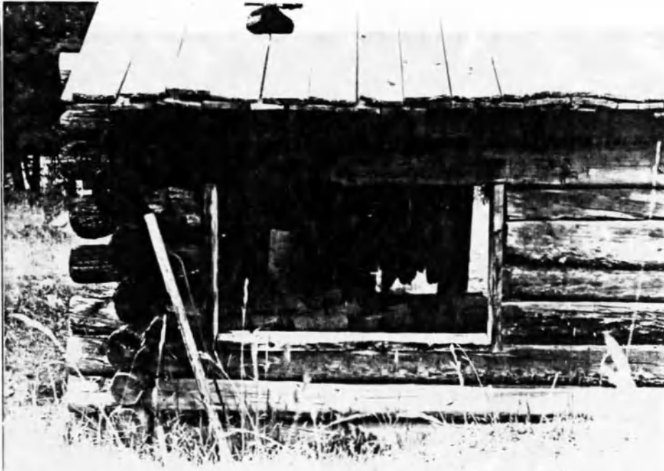
Figure 73: A view of Liberty's blacksmith shop after stabilization and removal of the shed and forge.
