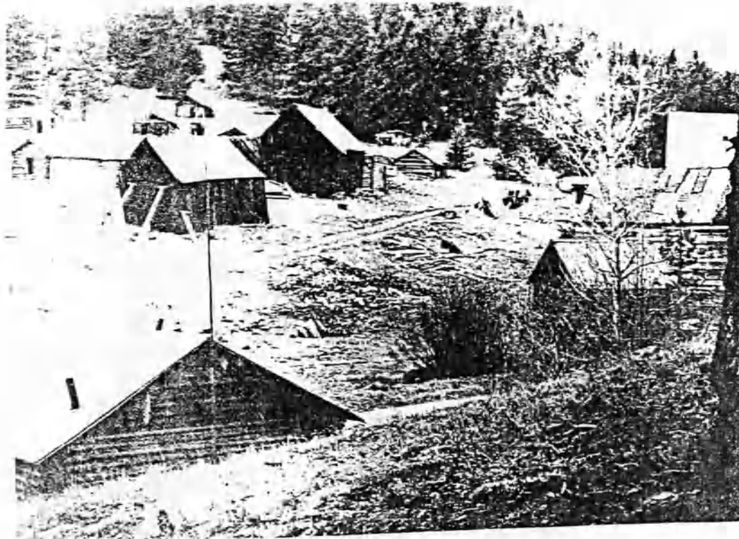
Figure 9: View of Garnet in 1971 (Hammond 1983). Notice the presence of supports on the building seen in the middle of the photograph.
