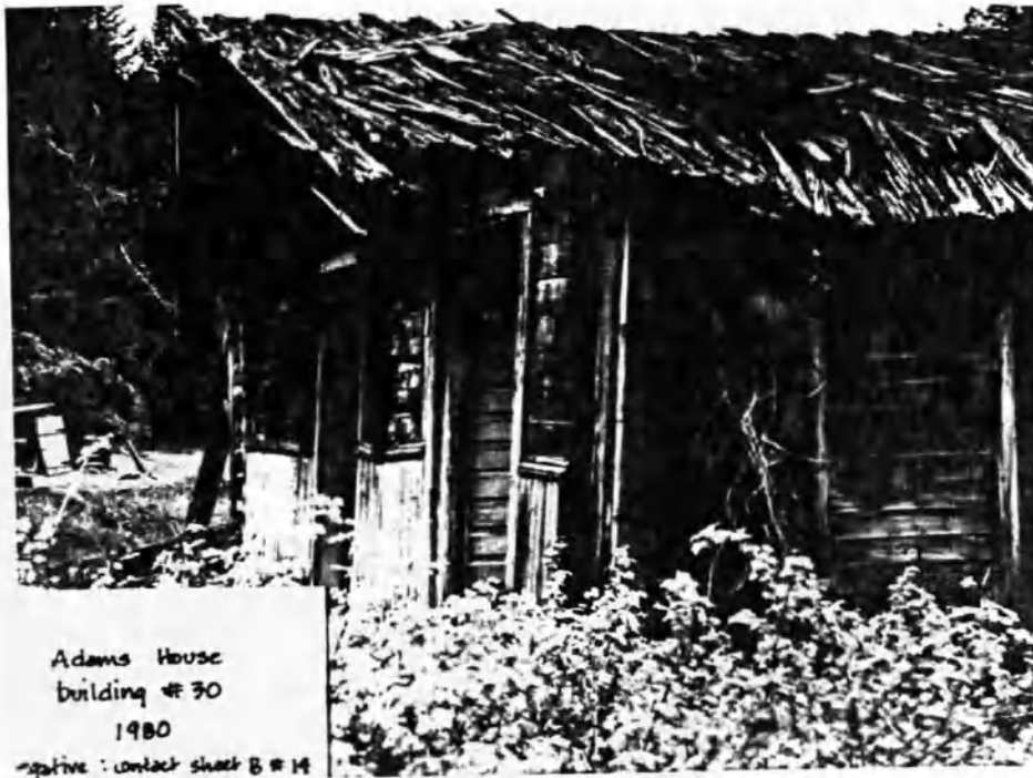
Figure 17: A 1980 photograph of the Adams family house. Notice the deterioration of the roof and the sagging walls.
