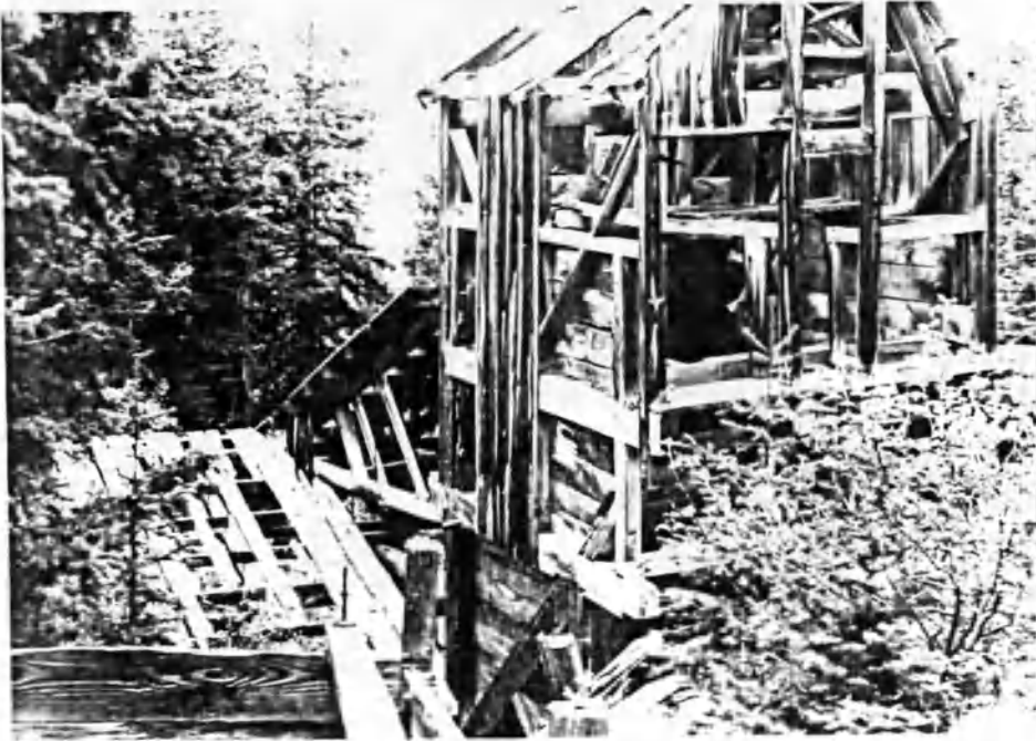
Figure 28: A photograph of the east side of the Mountain View mill.
