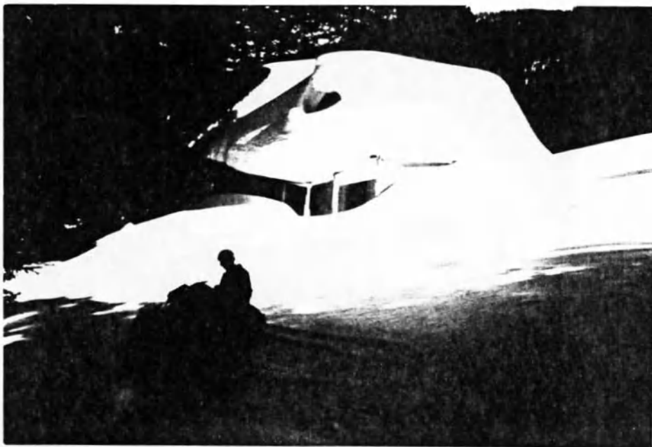
Figure 103: Although ten years earlier, there is a considerable amount of snow on the Dalhberg house. The continued stress of such heavy snow falls year after year cause some buildings to collapse.
