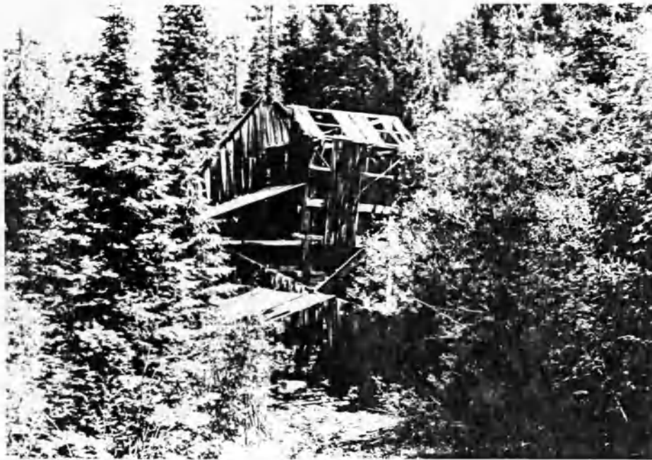
Figure 29: A photograph of the Mountain View mill facing northeast.
