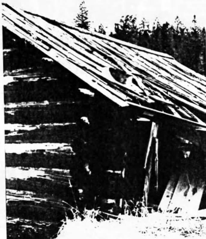
Figure 72: A photograph of Billy Liberty's blacksmith shop prior to restoration (BLM photograph). Notice the metal pipe end extending above the roof.
