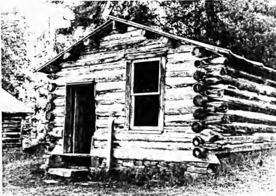
Figure 90: The photograph of the cabin shows a rather large window, but does not show it is the only window in this structure. Also note that this structure has barked logs, no foundation, and a dirt floor
