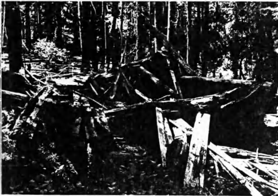
Figure 49: A cabin located down the hill from the Mountain View mill. Notice the deterioration or rotting of the logs in the structure.
