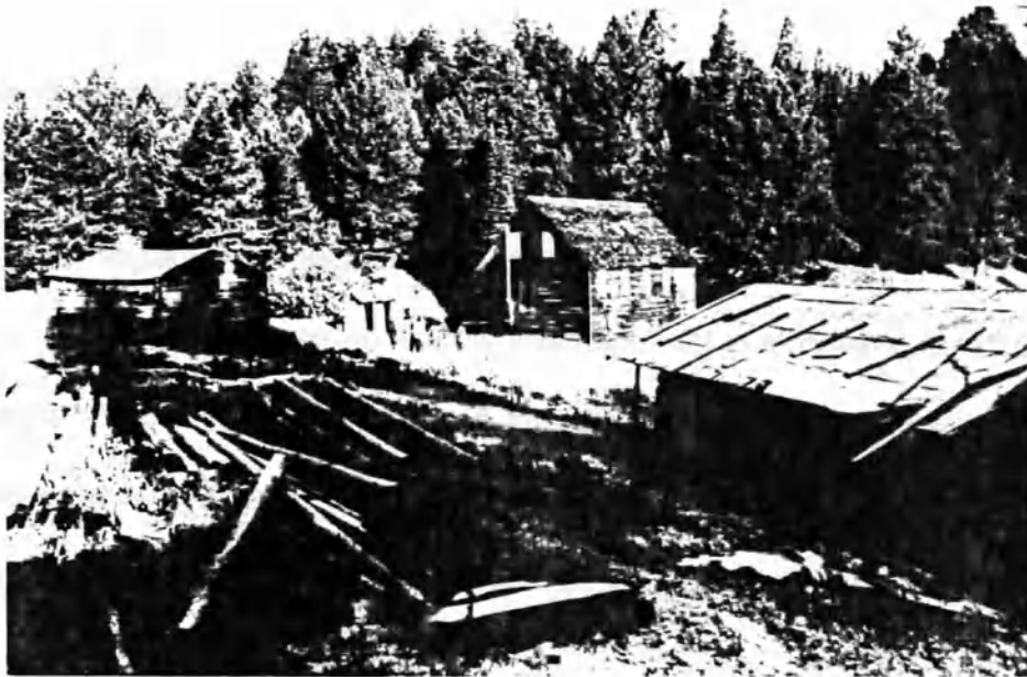
Figure 98: An undated photograph of the Honeymoon cabin. Notice the absence of roof planks, but the presence of tar paper
