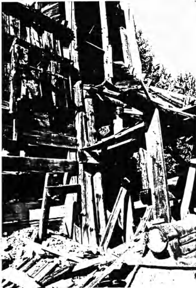
Photograph 20. Ore chute.
