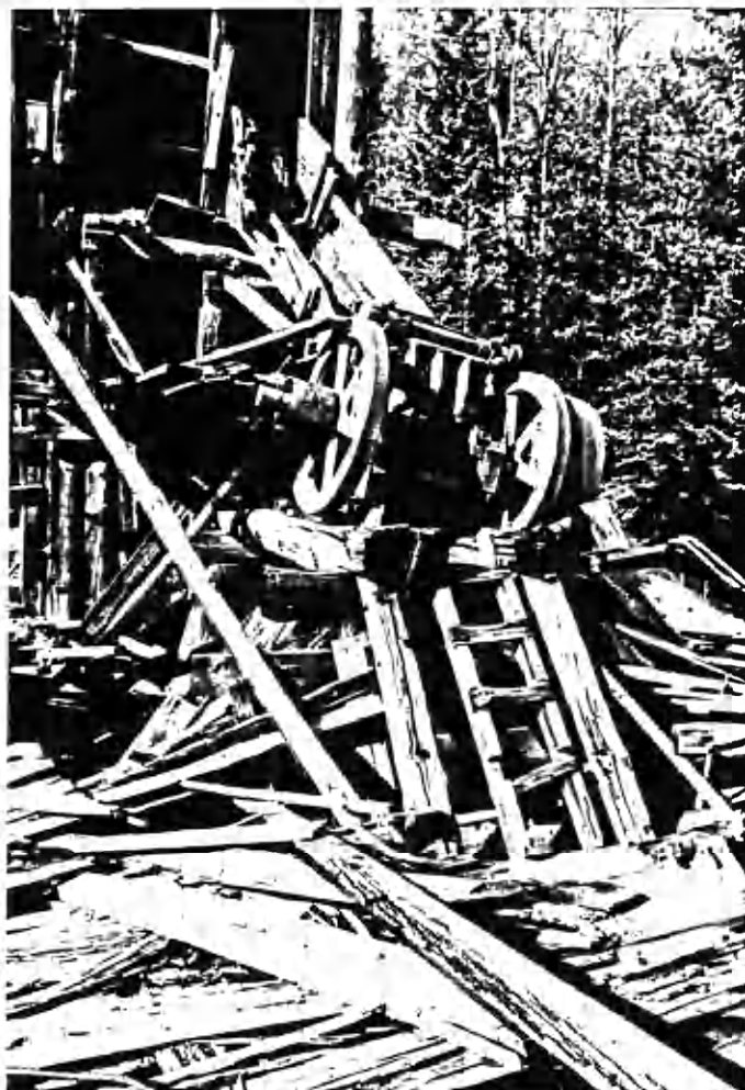
Photograph 22. Jaw crusher.
