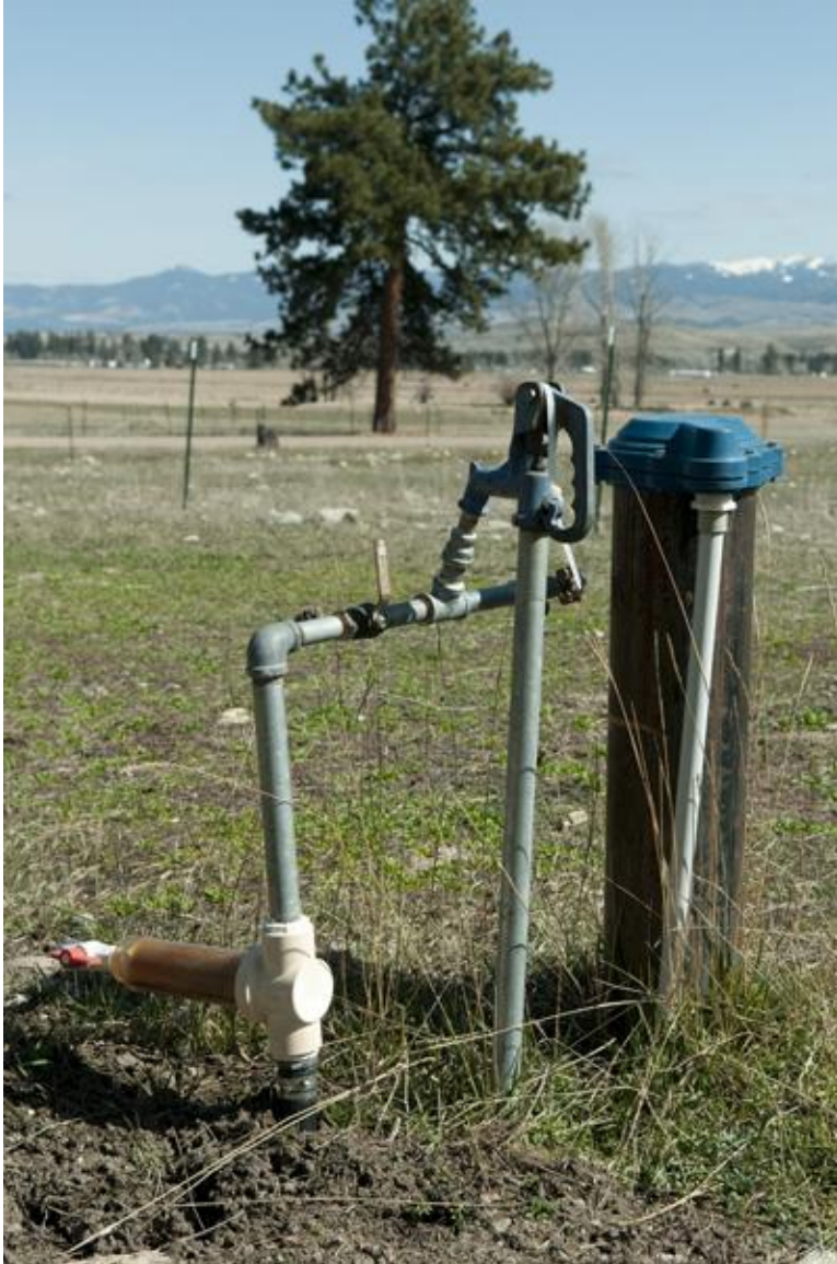
A new well awaits another house south of Hamilton.
