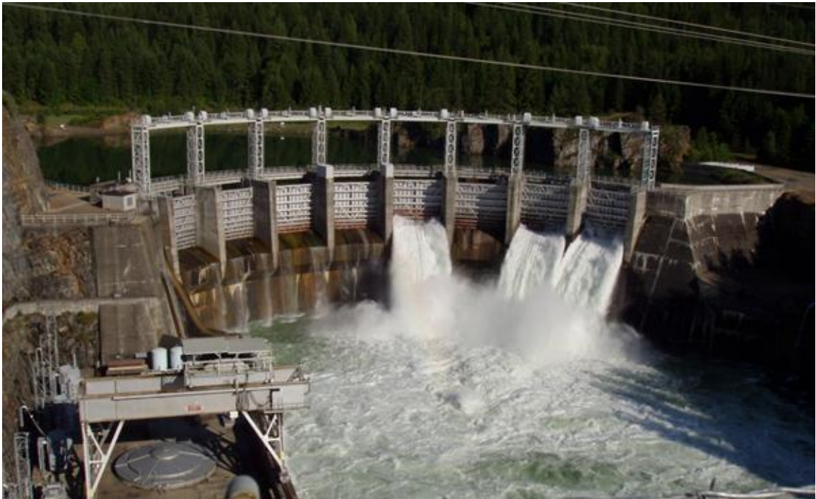
The Noxon Rapids Dam sends Clark Fork River water through three of its eight turbines.
