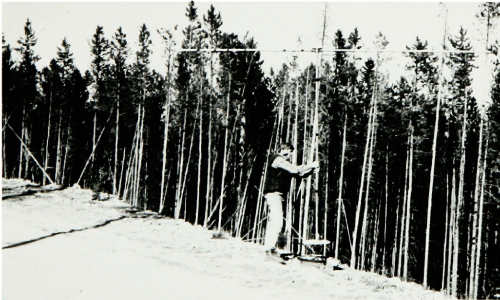
Fig. 9.--Eight element Yagi for ground telemetry.
