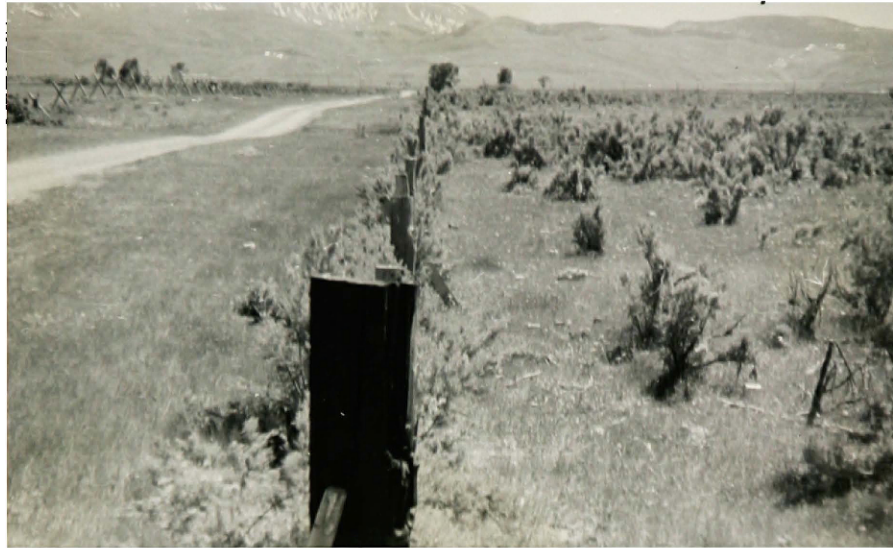
FIGURE 17A RELICT ROAD RIGHT-OF-WAY IN OLD SAGEBRUSH STAND NEAR DILLON
