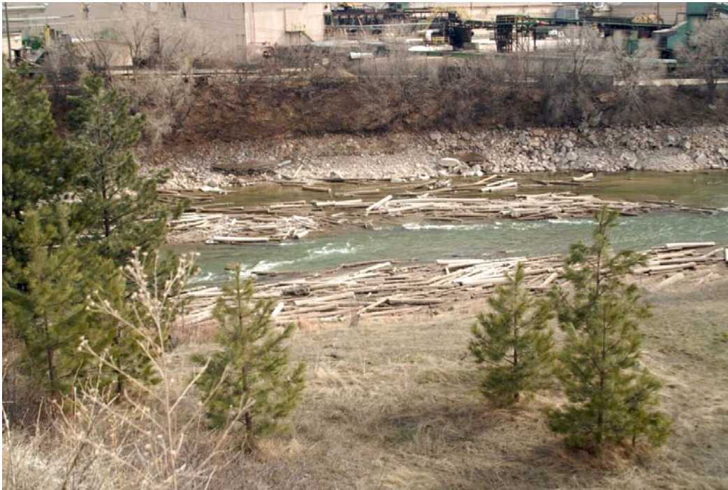
Figure 34. Lower BFR flowing for the first time since 1907 conversion to reservoir. Distinct sediment and vegetation banding shows phased reduction in base level, starting in 2006, and recently completed by the coffer dam breaching on March 28, 2008 (Photo taken 4/8/2008)
